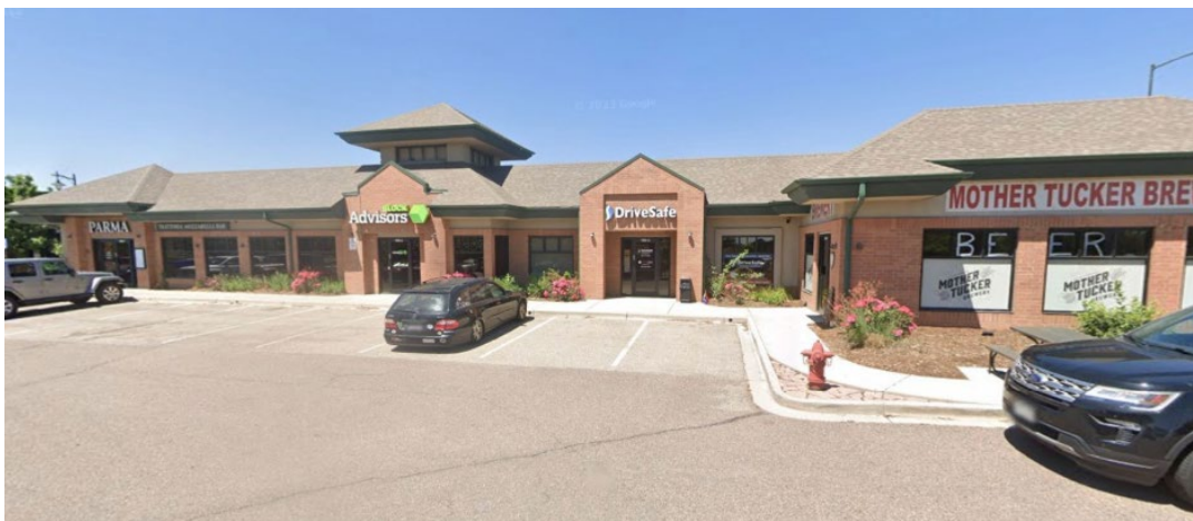
Current image of one of three existing commercial buildings.
