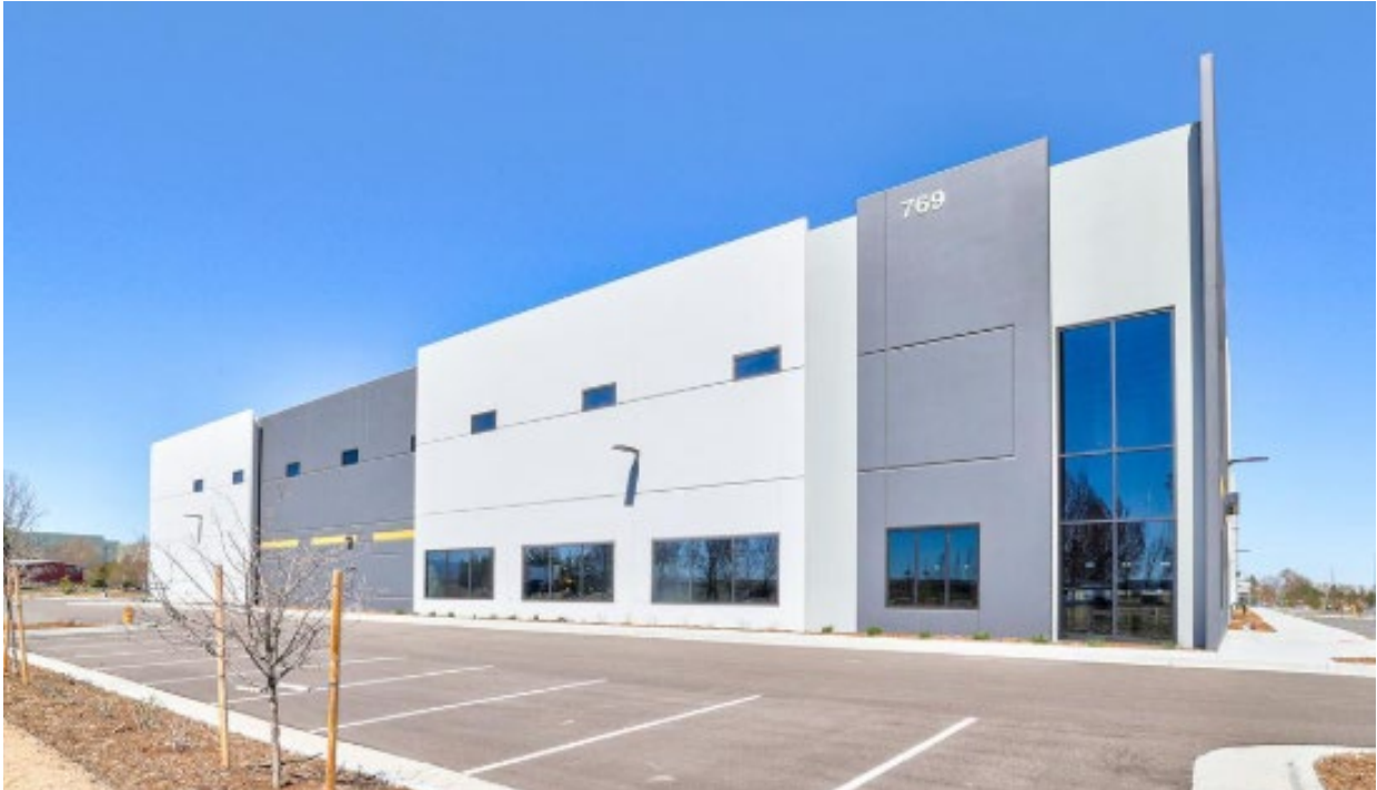
Example of Tilt-Up Concrete Construction facing Dillon Road at 769 CTC Blvd in the Colorado Technology Center within the Industrial Zone District
