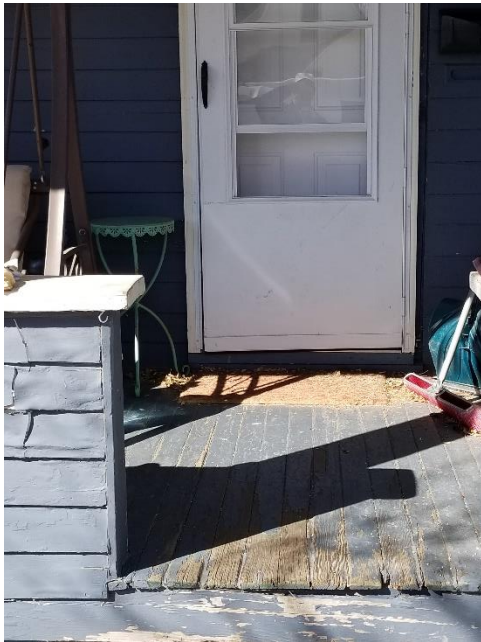
front porch siding, trim, floor, door
