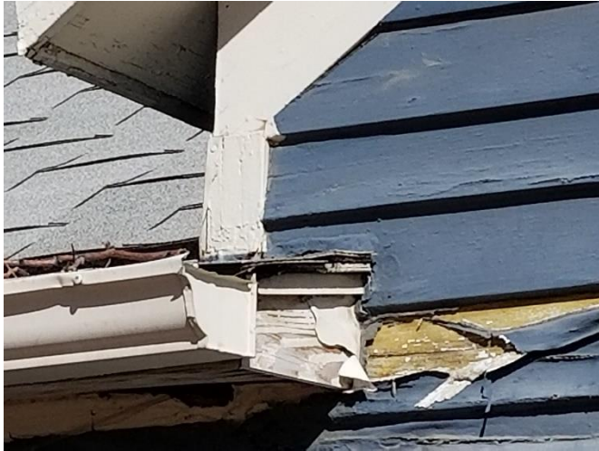
patch, sand, prime, paint
