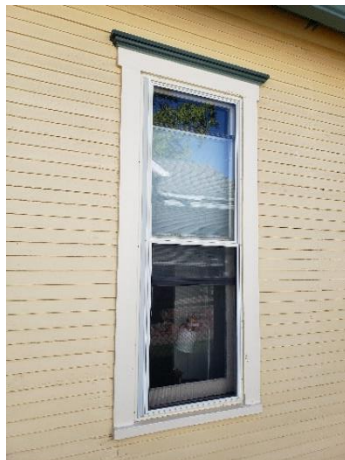
Wood window with aluminum frame storm window and screen.
