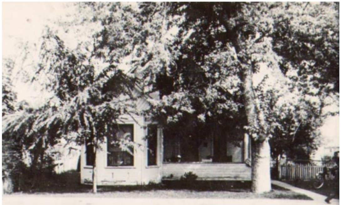
1950 Boulder County Assessor card photo of 1016 Main and floorplan.
