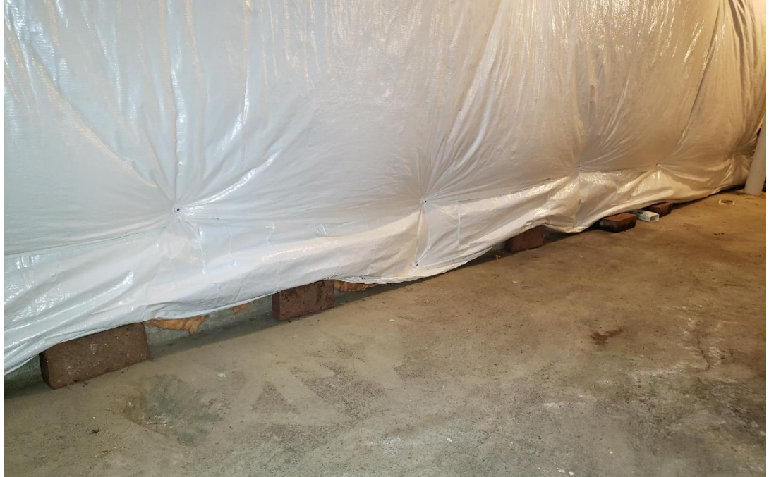
The concrete retaining walls are minimally exposed as they are covered by insulation.
