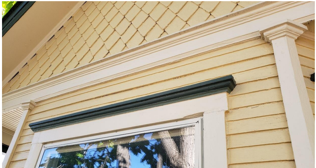
Decorative painted wood trim is found at the windows, doors, corners, and gable ends.
