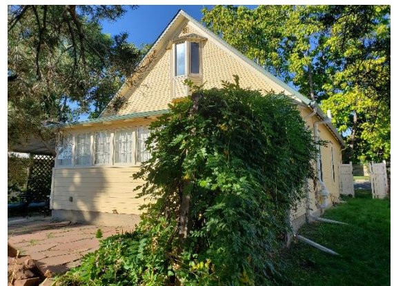
Vines growing on trellis structure.
