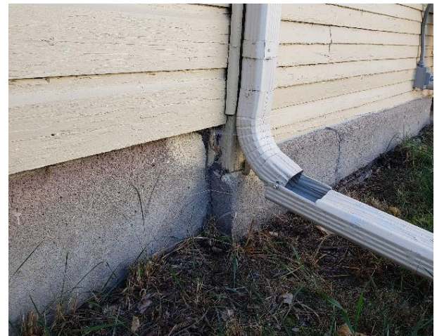
A jog in the foundation shows the concrete face over the original stone foundation (right) relative the concrete foundation of the east addition (left).
