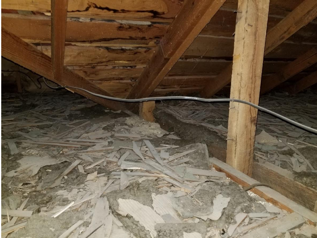
Attic framing, sheathing, debris
