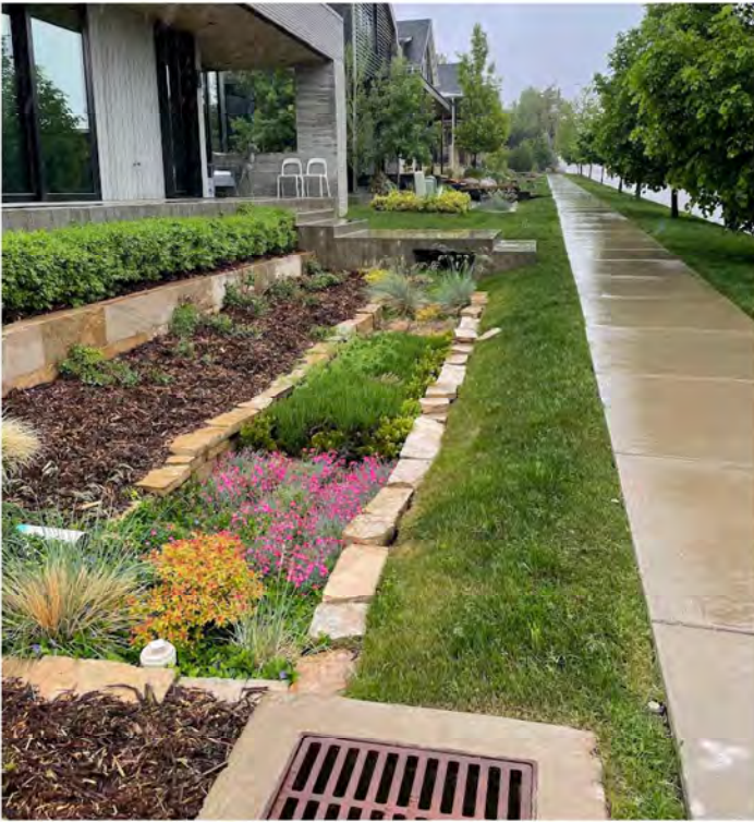
Photograph BR-1. This bioretention area treats runoff from the roof and lot, while serving as an aesthetically pleasing landscape feature. Photo: Wright Water Engineers.
