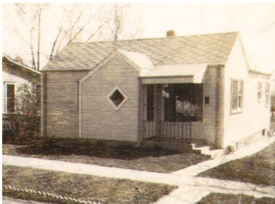
Boulder County Assessor photo from 1956 showing new vestibule addition.
