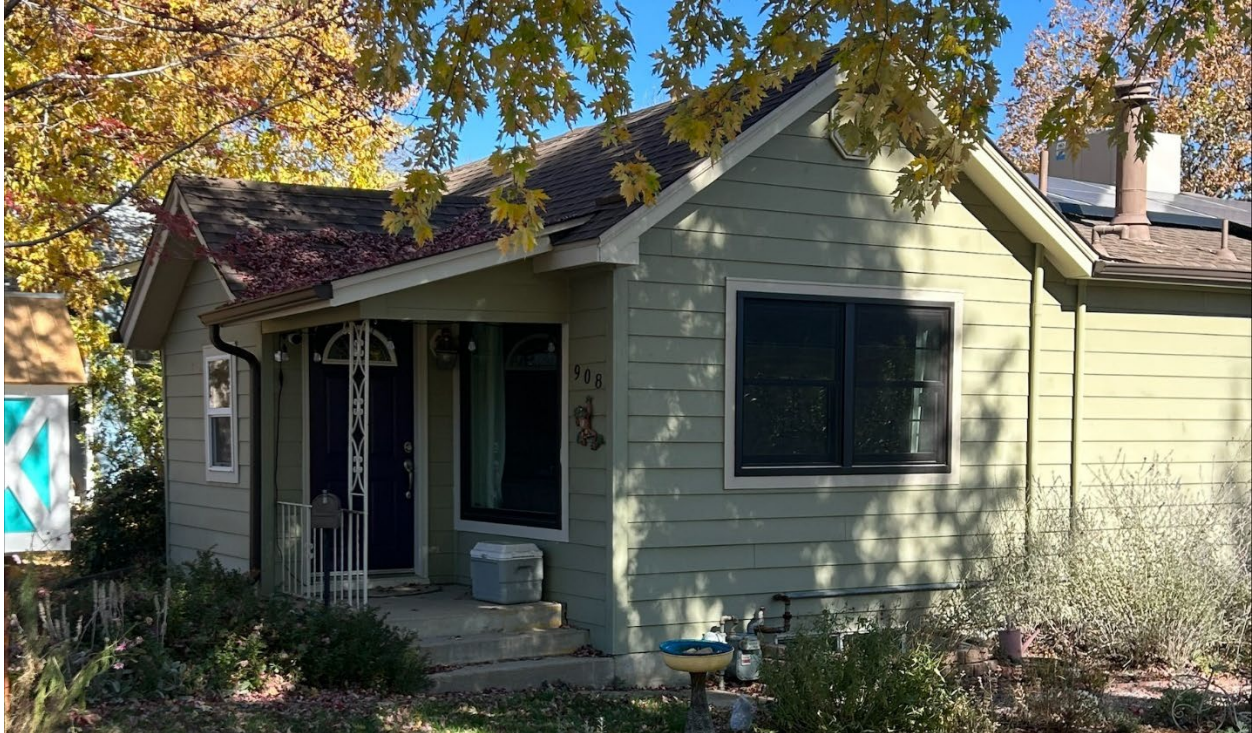
Current photo of 908 Garfield Avenue, October 2025
