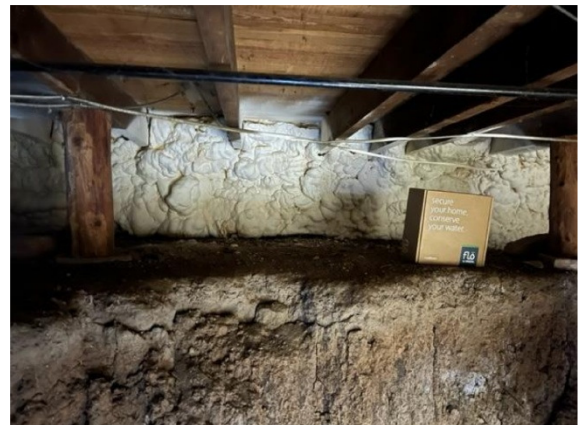
Figure 10: Logs under individual joists
