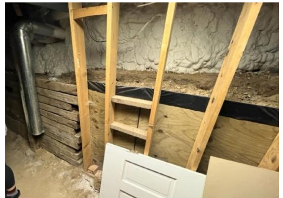
Figure 3: Interior of perimeter Foundation and wood cellar walls
