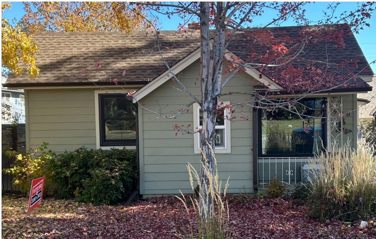
Current photo of 908 Garfield Avenue, October 2025
