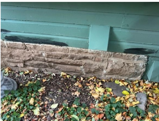
Figure 2: Exterior foundation with timber
