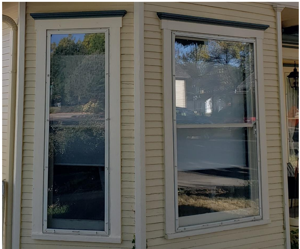
Double-hung wood windows with aluminum frame screen windows.
