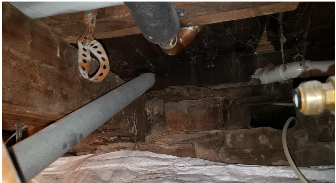
The foundation is minimally exposed as it is covered by insulation. The original foundation appears to be stone.
