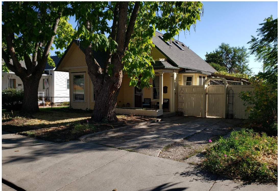
2024 View from the Southwest
