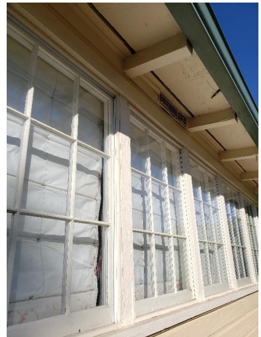
Exposed painted rafter tails at the east addition.
