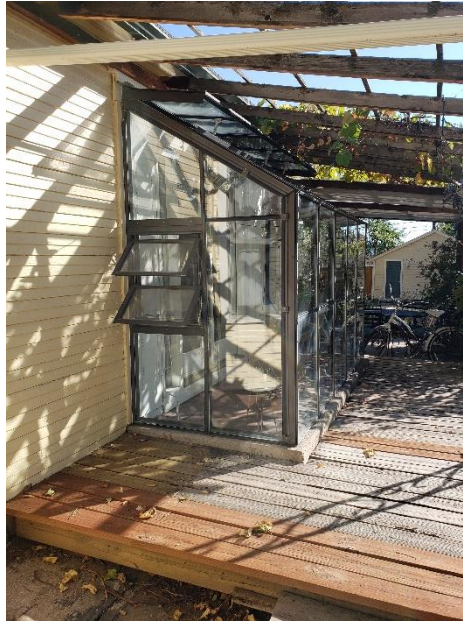
Greenhouse attached to the south of the house.
