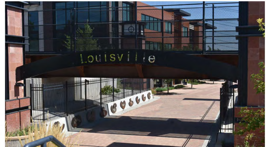
Louisville Bridge Source: DesignWorkshop
