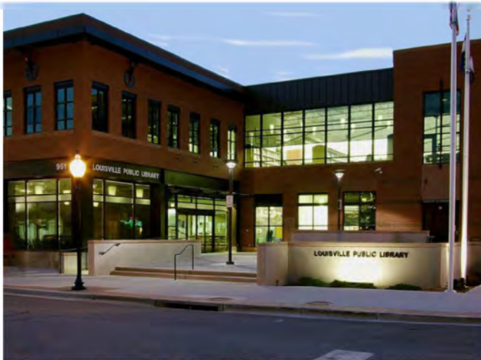
1 Louisville Public Library (Source: Louisville Public Library)
