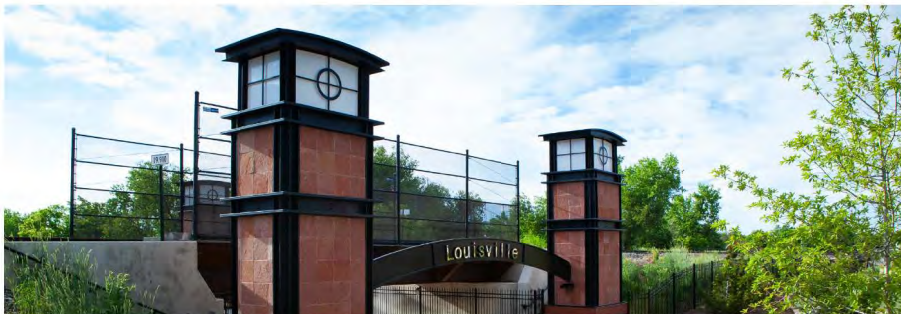
South Street Underpass Source: City of Louisville
