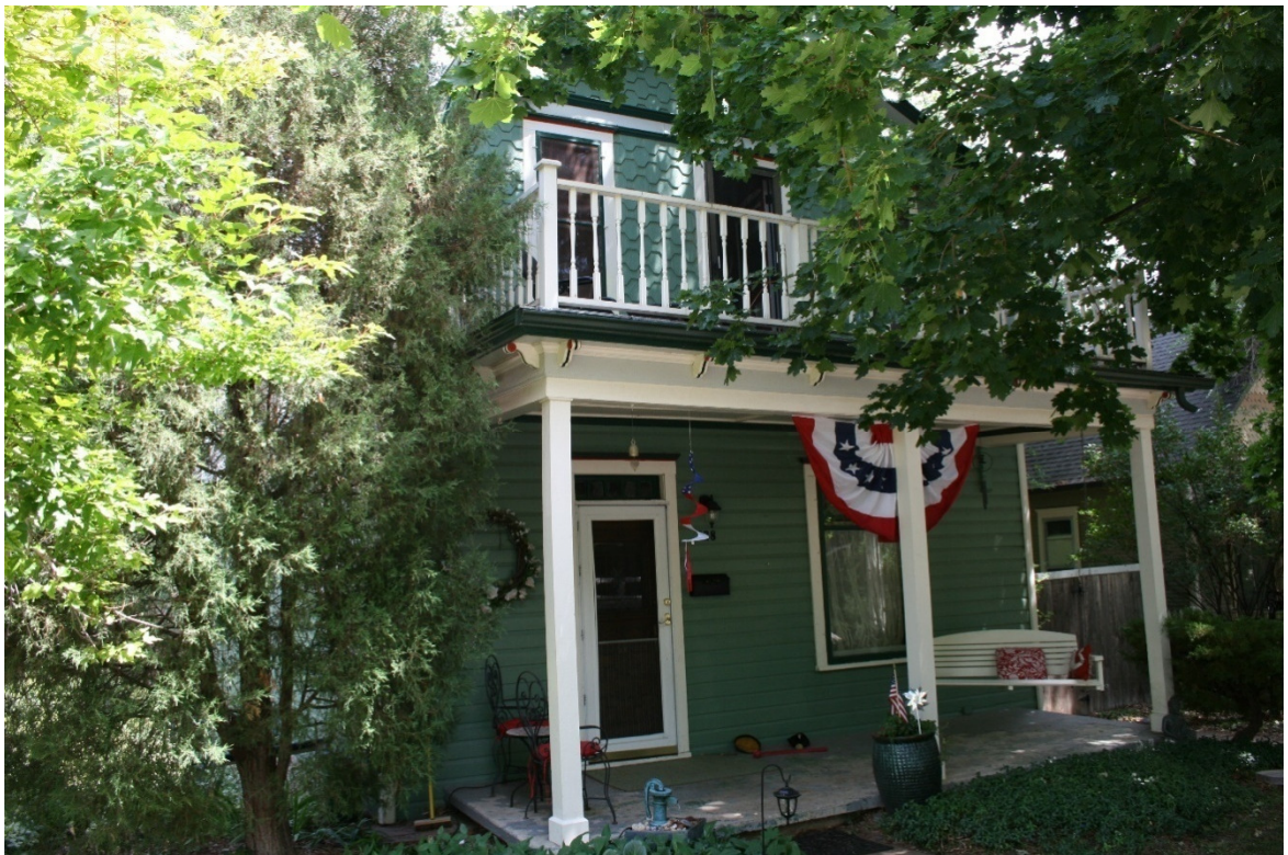
728 Grant Avenue, northwest elevation– 2013 photo
