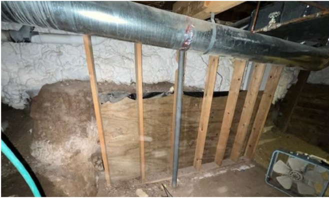
Figure 12: Wood retaining wall
