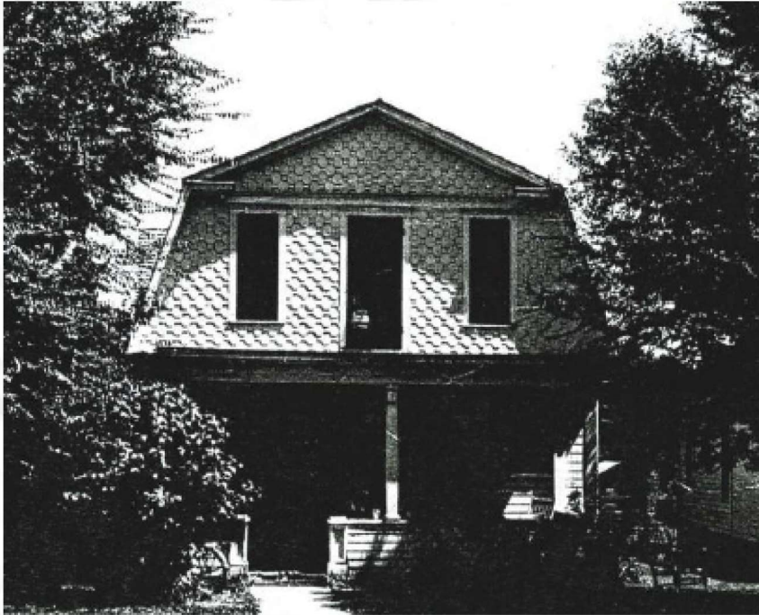
Photo from 1948 Boulder County Assessor Card
