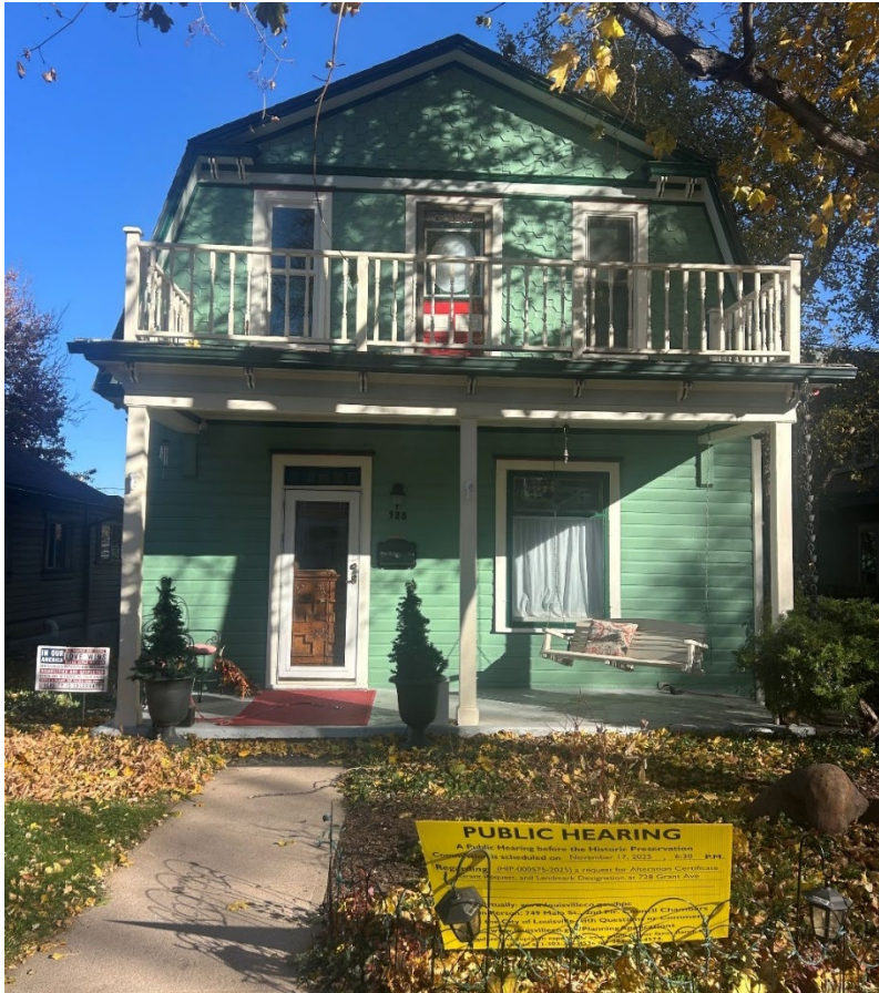
Current photo of 728 Grant Avenue, November 2025
