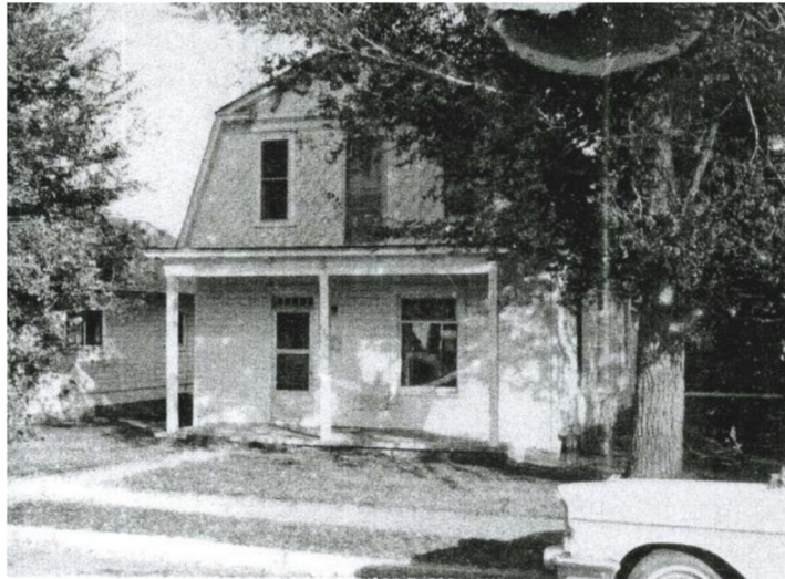
728 Grant Avenue, west (front) elevation – 1978 Boulder Assessors Card
