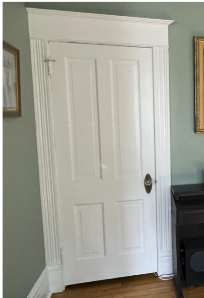
image 3 – original interior door 1 st floor – 3.5.1
