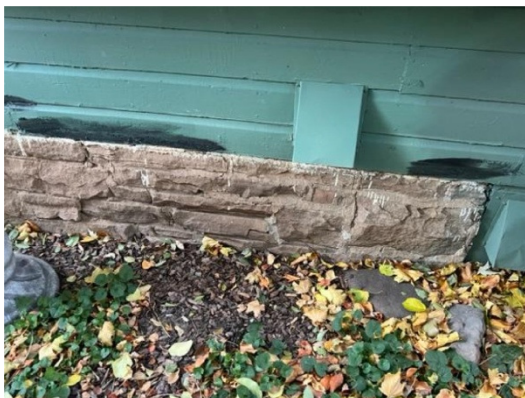
Figure 2: Exterior foundation with timber
