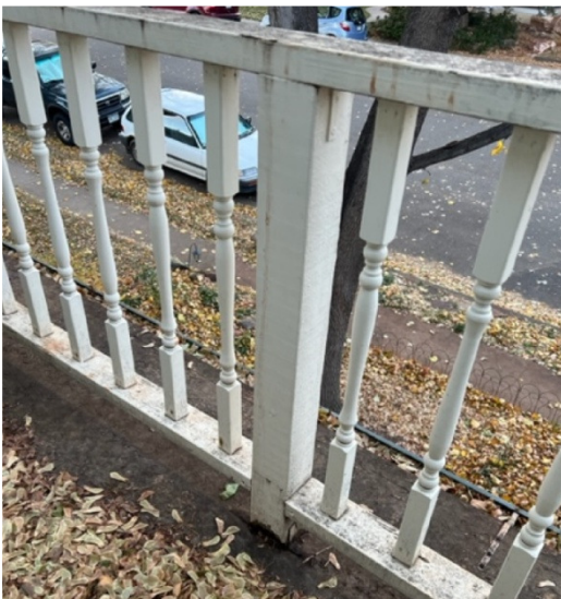
Figure 4: 2 nd Floor Deck Rail
