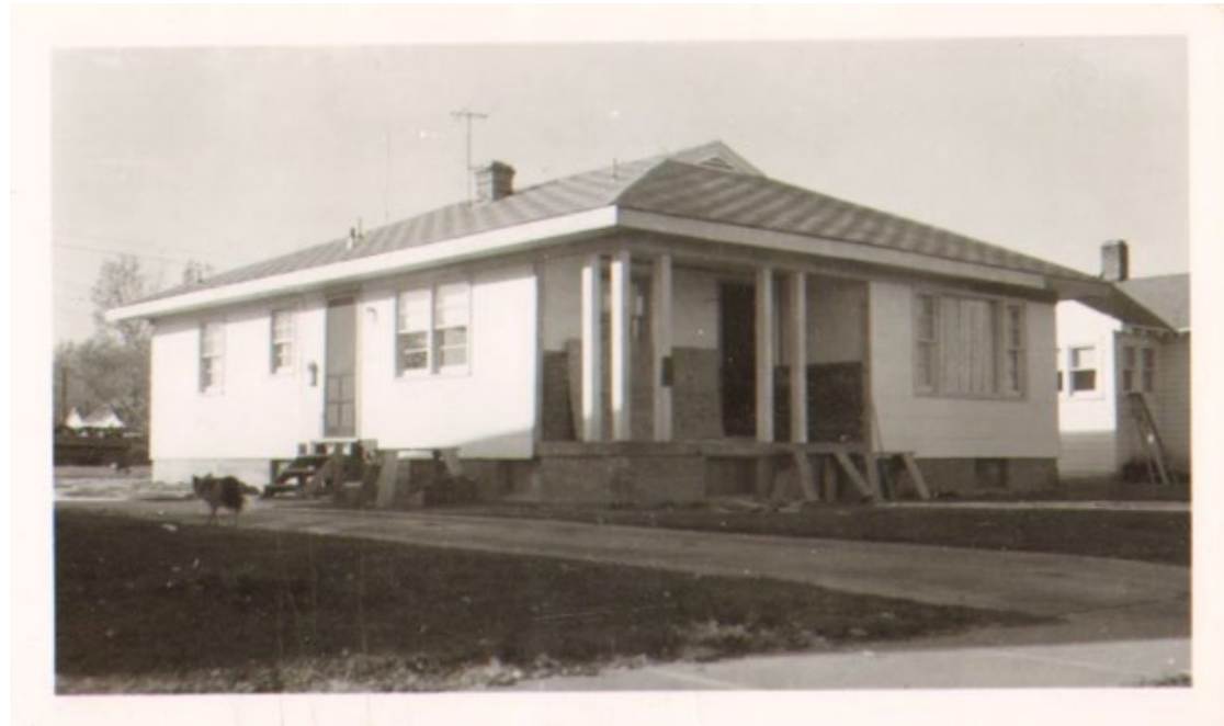
Photo of 517 La Farge Avenue from the Boulder County Assessor card from 1952.
