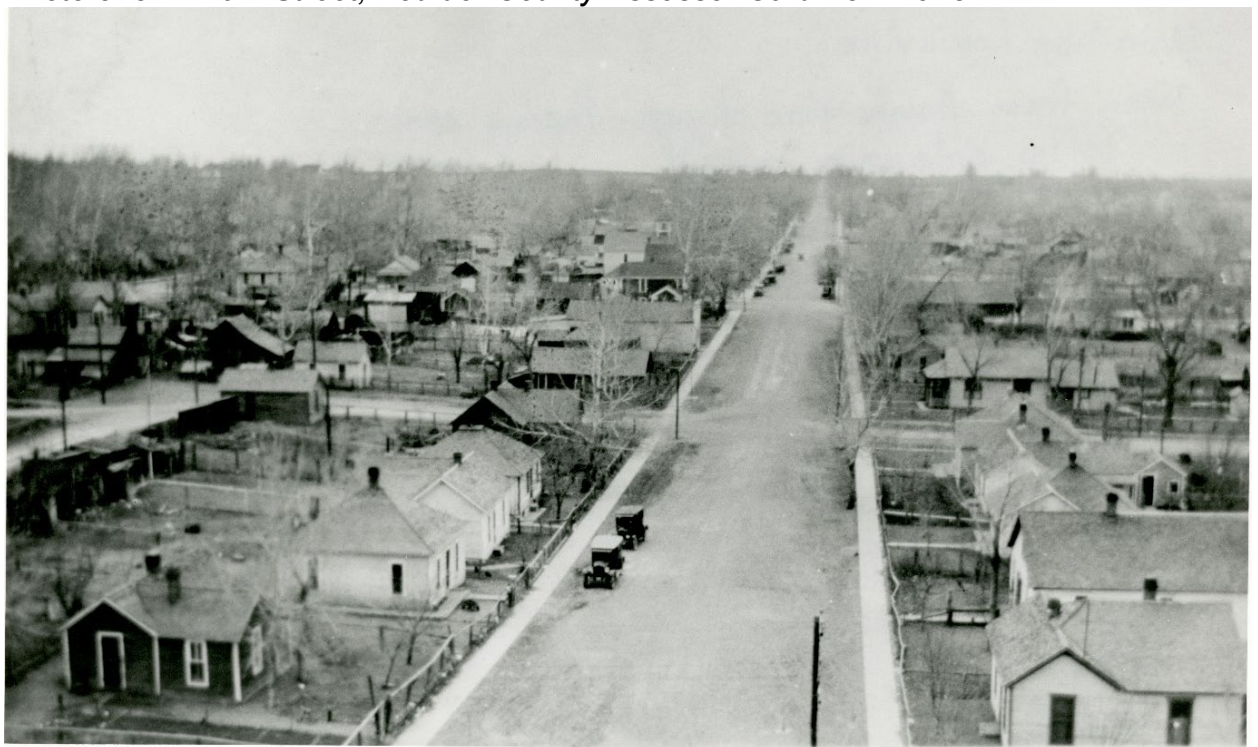
This undated photo taken from the top of the Acme Mine dump shows Main Street (Second Street) heading north. The house in the bottom right corner appears to be the location of 524 Main today. Photo is likely c. 1911-1928.
