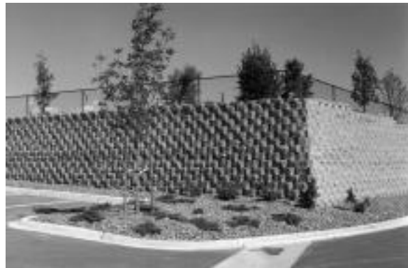
6.1.A - AVOID RETAINING WALLS IN EXCESS OF 30"
