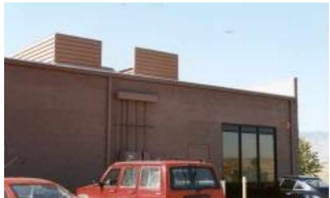
4.4.C - RTU's NOT PROPERLY SET BACK FROM BUILDING EDGE
