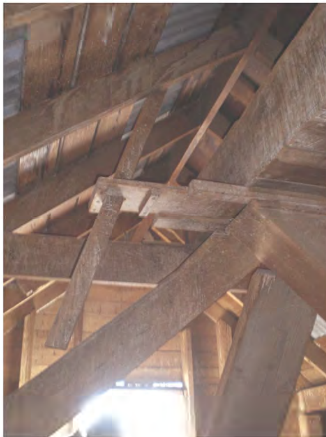
Fifth Floor - Operating mechanism to control grain entering the grain bin chutes
