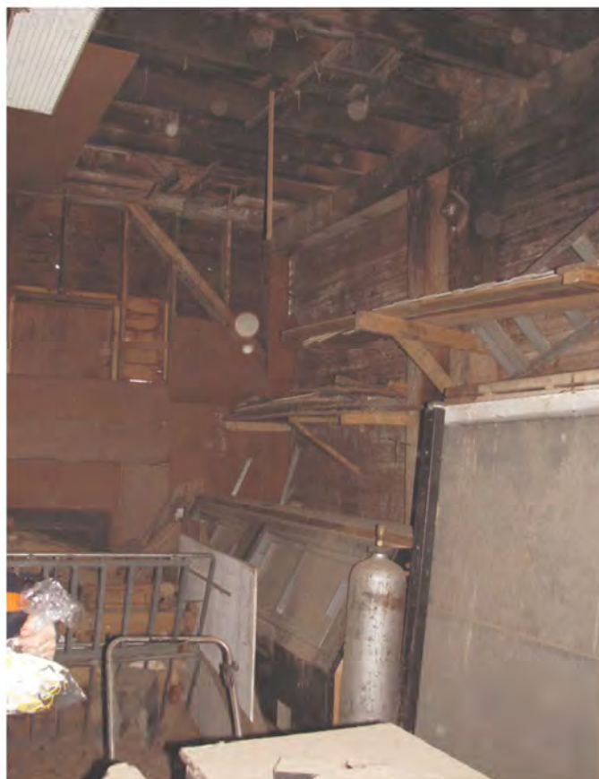
First Floor - Tower Level 1 looking at southeast corner
