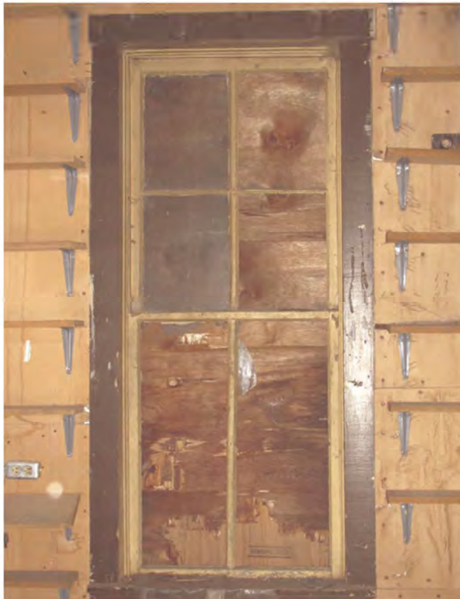
Interior side of window 7
