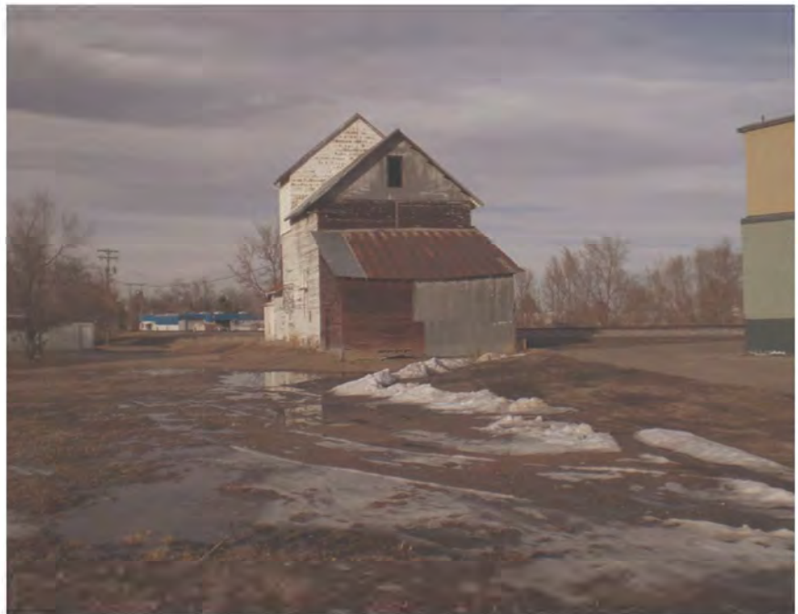
Looking north at the Grain Elevator with the railroad tracks and warehouse on the right
