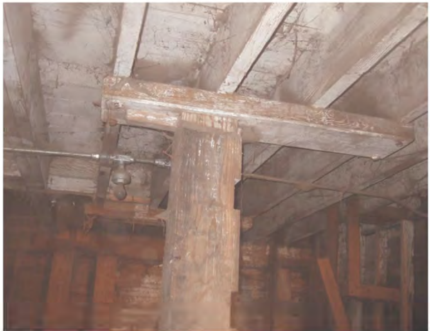
Section 3: First floor framing, wood post and 'corbel'
