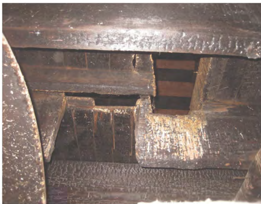
Section 3: Sixth floor mezzanine framing with notch
