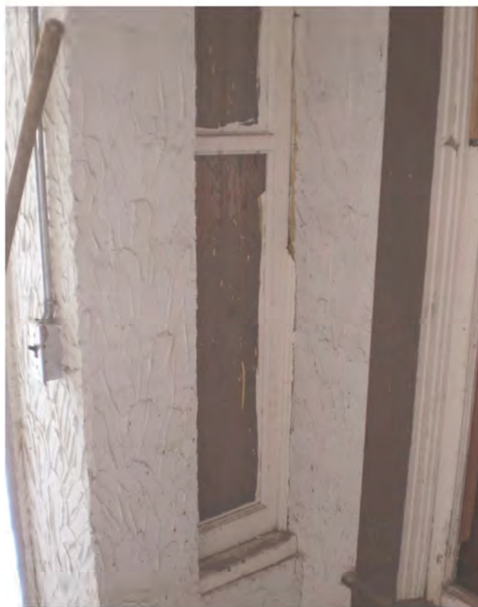
Window 2 interior side
