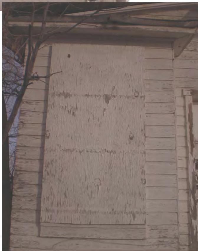
Exterior side of window 1
