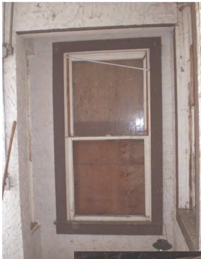
Interior side of window 1
