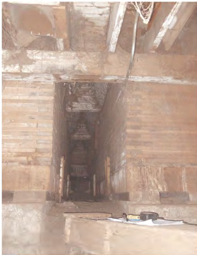
Section 3 & 4: First floor framing beam and joists along grid 4; flared bins wall beyond along building centerline
