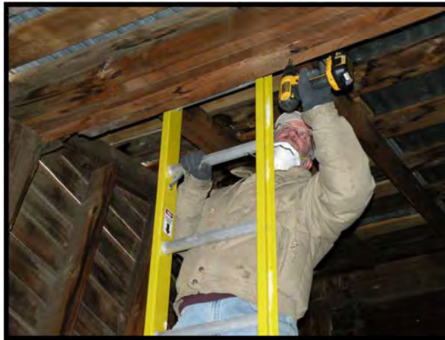
Figure 1. Removing a sample for species identification from a built-up beam, Section 5, Storage Room.
