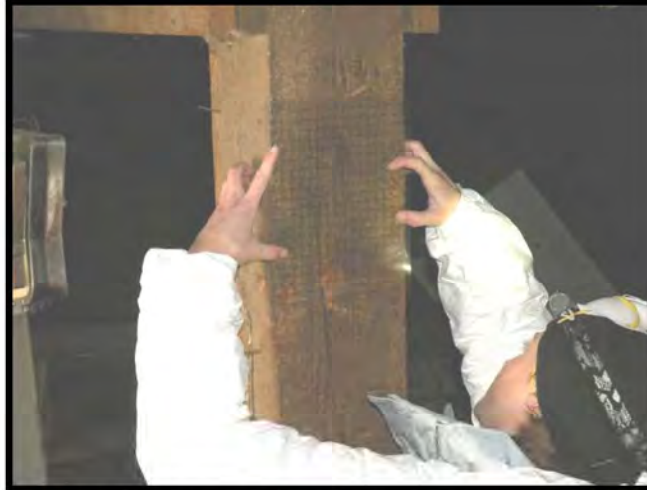
Figure 2. Measuring the slope of grain on a column with an acetate grid.
