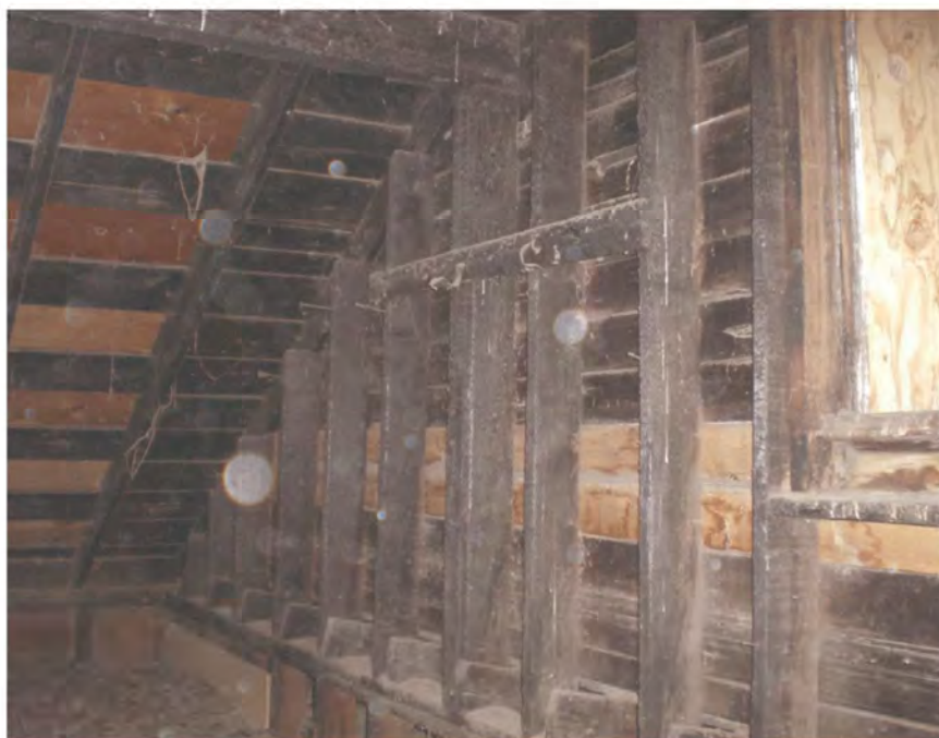
Second Floor - Looking west along north wall
