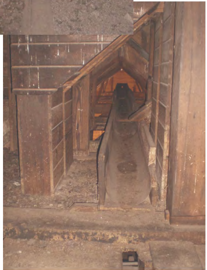
Sixth Floor - Chute to grain bins
