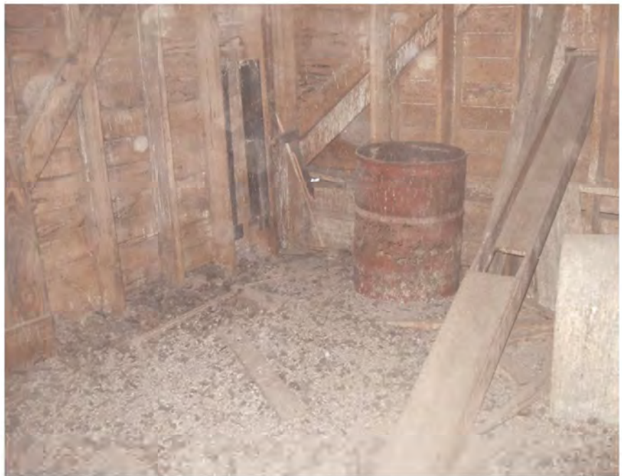
Section 3: Fourth floor exterior wall along grid 3 and grid A; 2x diagonal bracing lapped over wall studs
