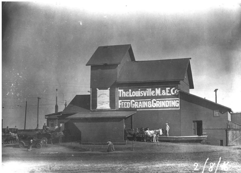
Louisville Grain Elevator, 2/8/1916, Louisville Historical Museum
