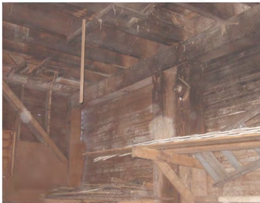
Section 3: Southeast corner of third floor framing bay
