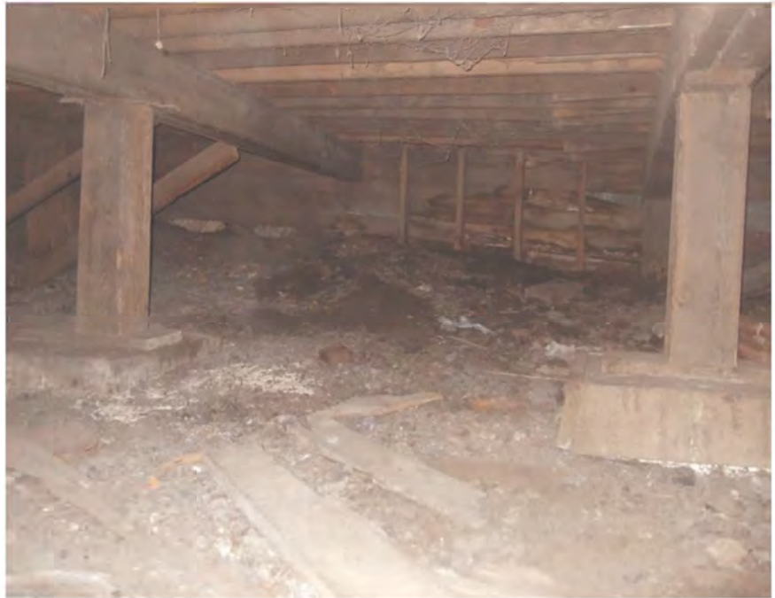
Section 5: First floor framing, looking south
