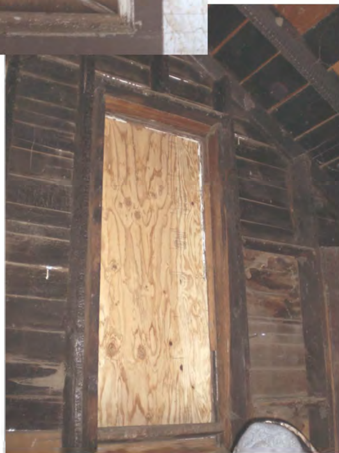
Window 9 interior side
