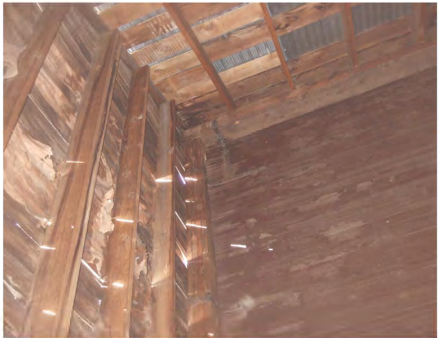
Section 5: Exterior wall studs along grid Z at grid 5; roof ledger along grid 5
