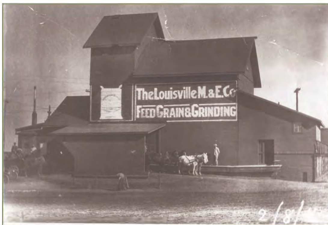
Photo of the Grain Elevator, 2/8/1914. Courtesy of the RFP from the City of Louisville
