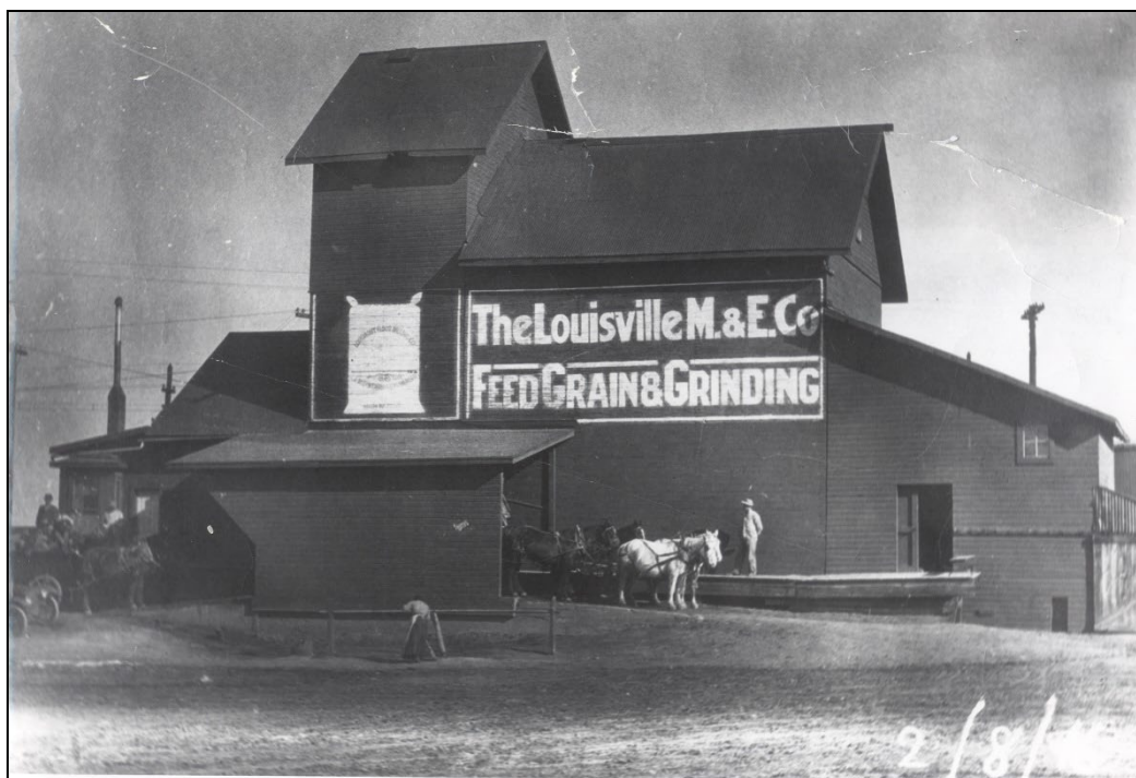
Louisville Grain Elevator, 2/8/1916, Louisville Historical Museum
