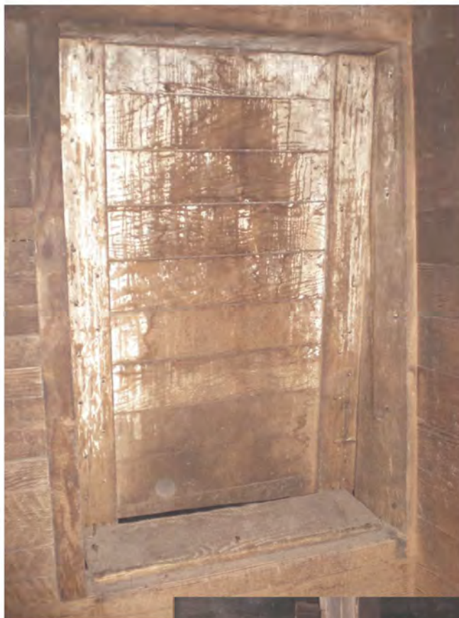
Third Floor - Access hatch into chute
