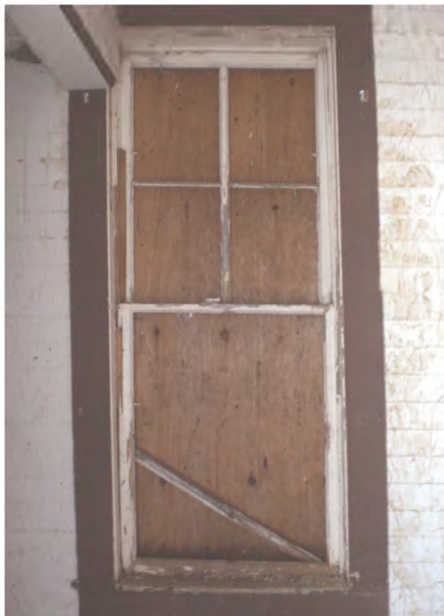
Window 8 interior side
