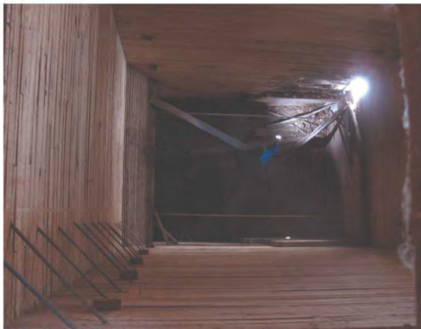
Fifth Floor - Looking down into Bin 5
