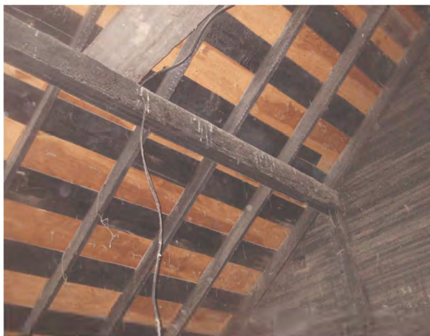
Section 2: Gable roof rafters over dropped purlin, looking south at grid 4
