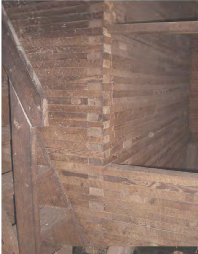
Third Floor - Chute 2 has been cut down while Chute 1 (on the left) continues up to the ceiling
