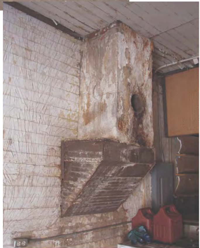
First Floor - Entry chimney on north wall
