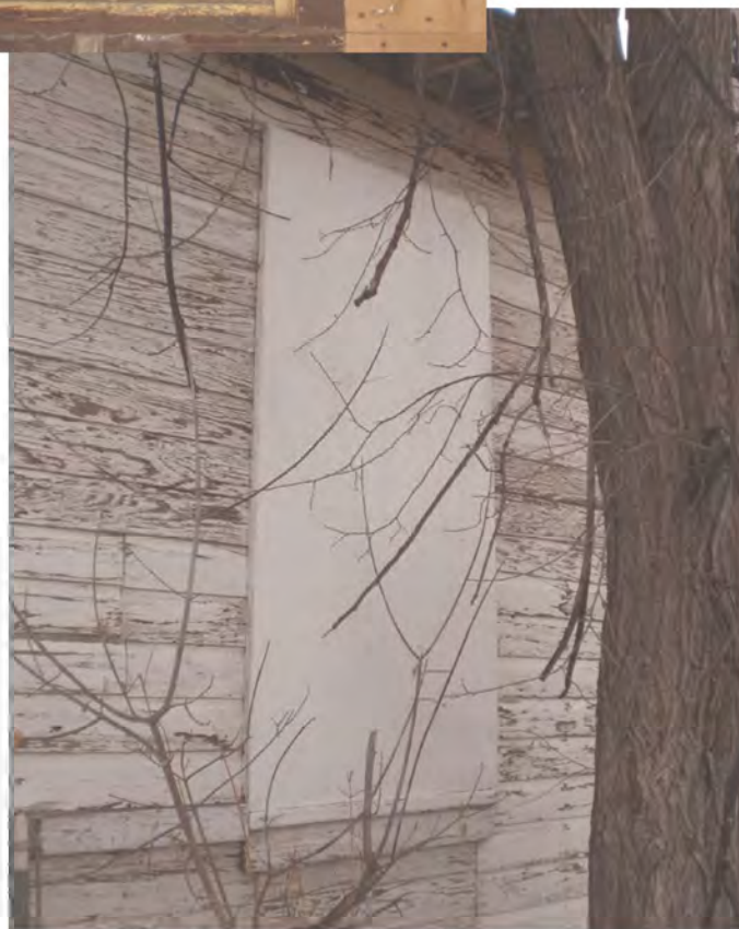
Exterior side of window 7
