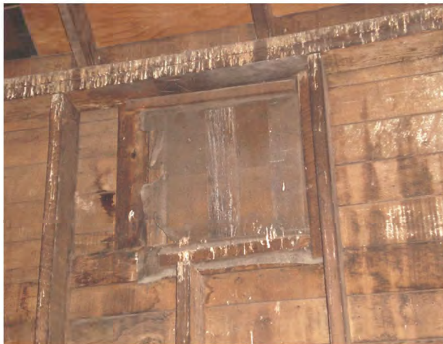
Window 10 interior side
