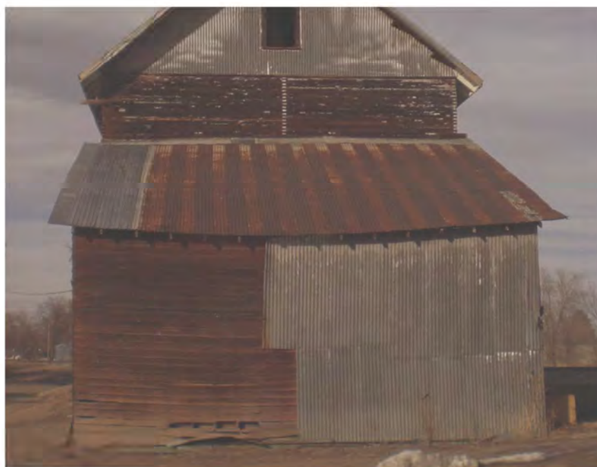
Corrugated metal roofing on Section 5
