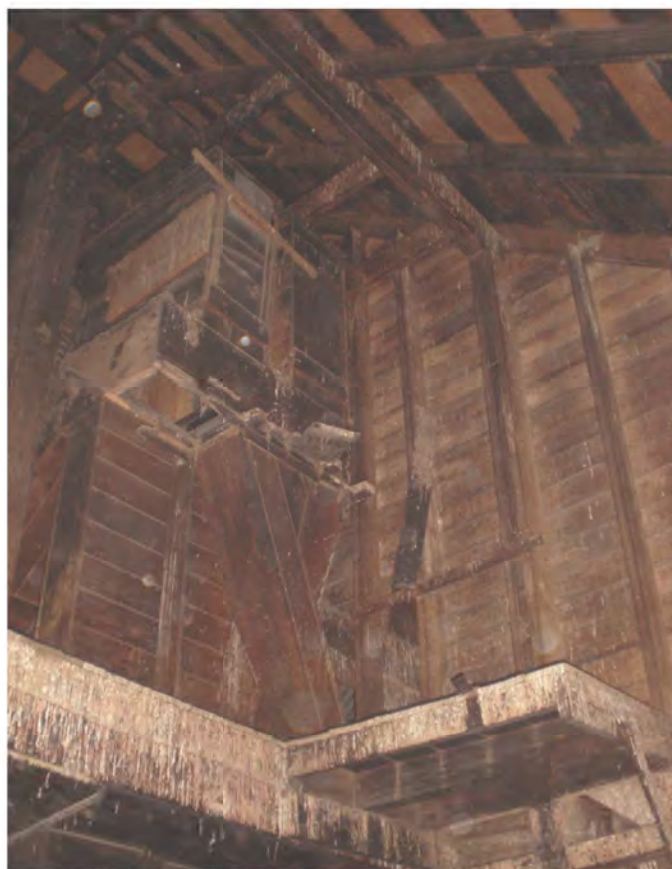
Fourth Floor - Looking up at chutes on the Sixth Floor
