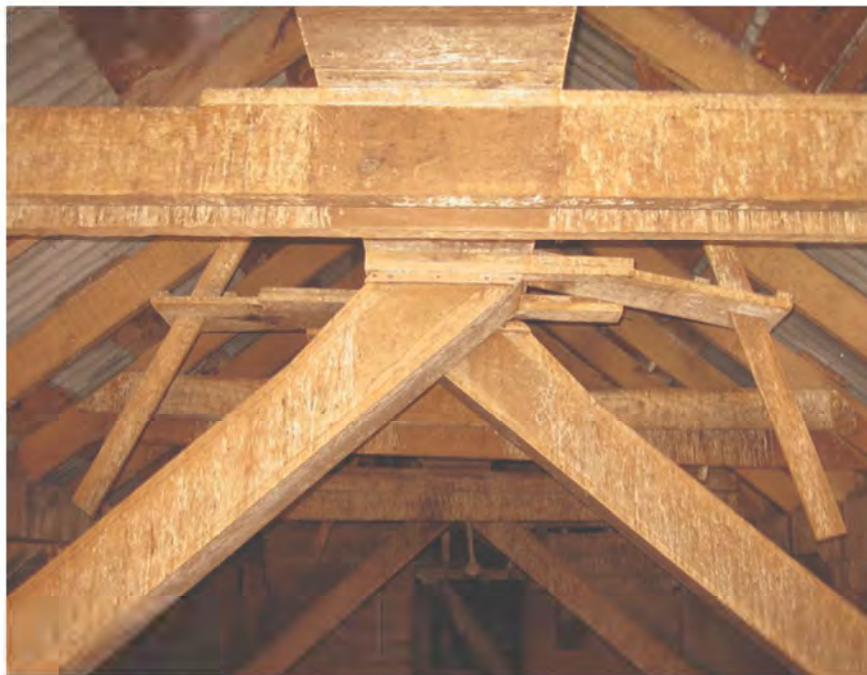
Roof structure and grain chutes in Section 4
