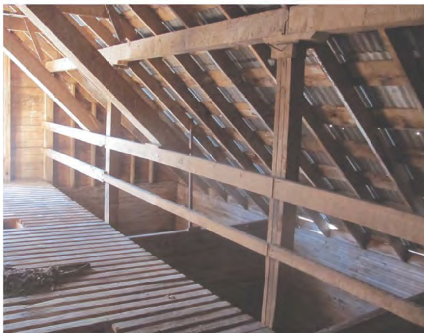
Fifth Floor - Bin catwalk and railing
