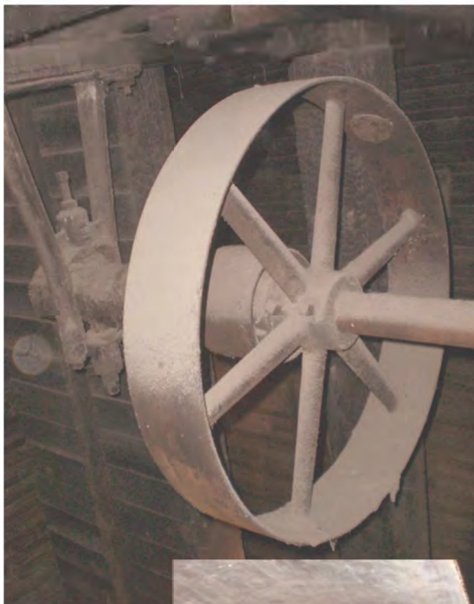
Elements of the conveying system on the third floor
