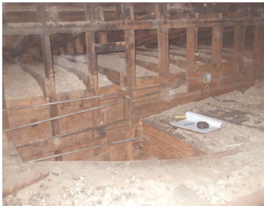
Section 1: Shed roof framing and flat ceiling framing, looking north at grid 2
