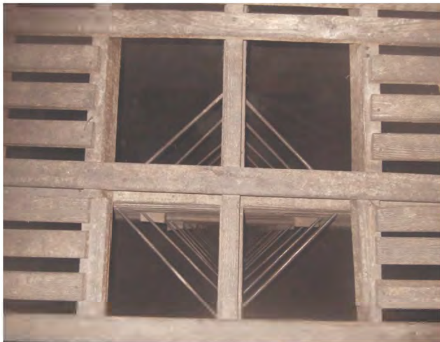
Looking down at the ladders leading from the fifth floor into the grain bins
