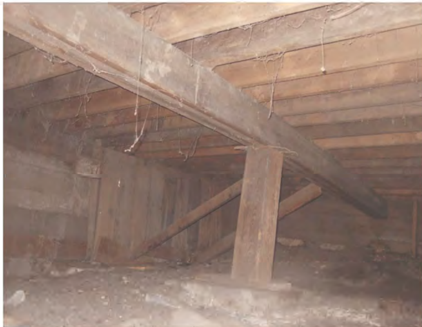
Section 5: Foundation wall along grid A and grid 6; crawlspace access opening remnant; diagonal bracing
