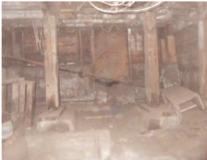
Section 3: First floor support posts and footings; foundation along grid A beyond
