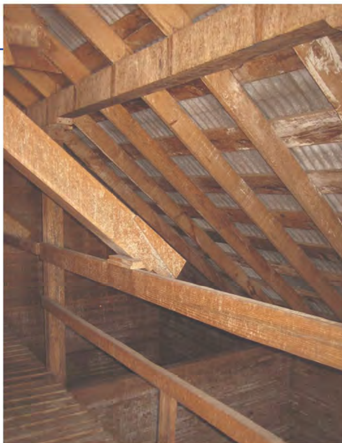
Section 4: Gable roof rafters over dropped purlin on east side
