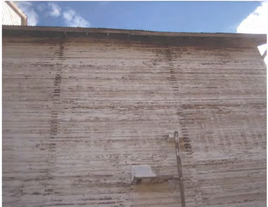
Section 4: Stacked-plank bin wall along west elevation, lapped plies at cross dividing wall corners
