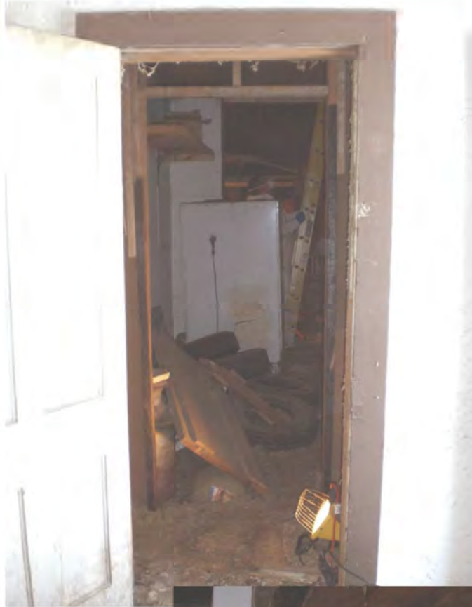
First Floor - Corridor looking south
