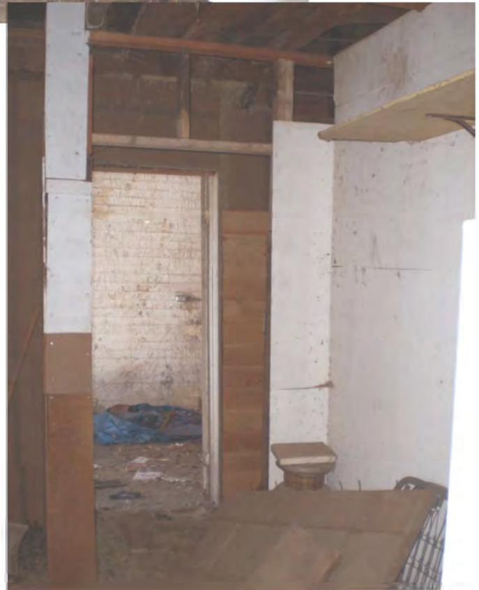
First Floor - Corridor looking north
