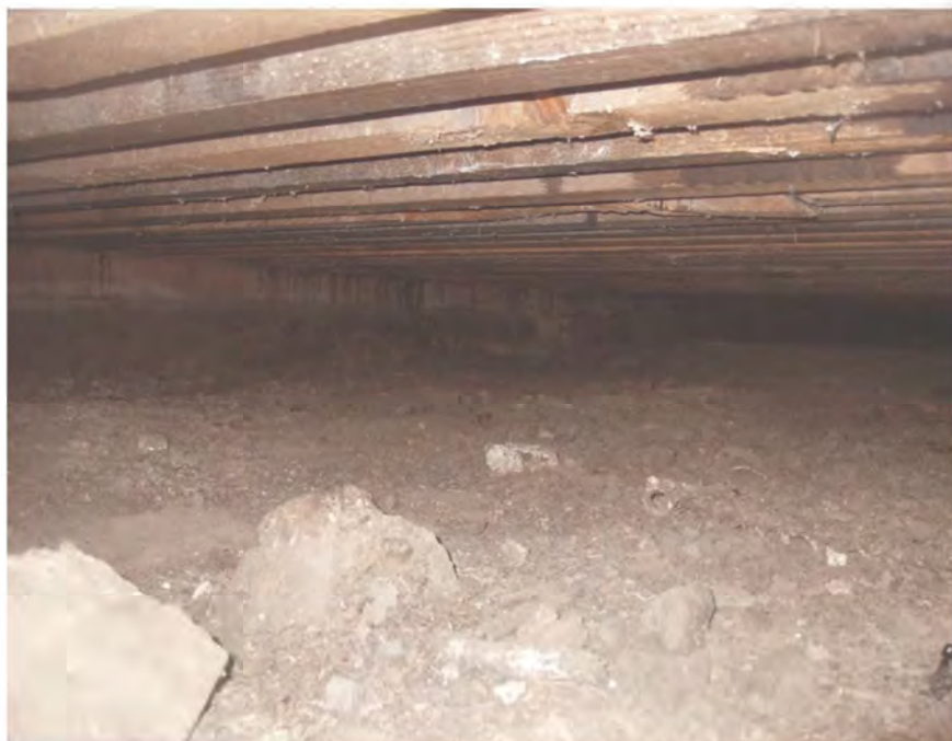
Section 4: Underside of Bin 1 floor framing
