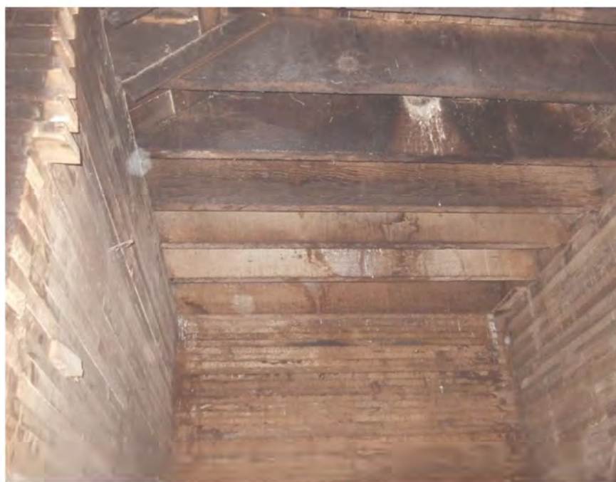
Section 3: Fourth floor framing; stacked-plank Chute 'partitions' below
