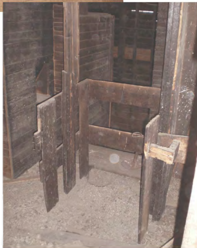
Third Floor - Track at original elevator shaft
