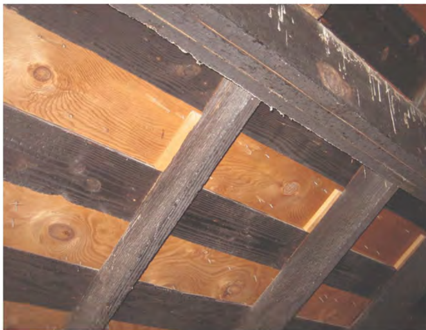
Section 3: Gable roof rafters over dropped purlin
