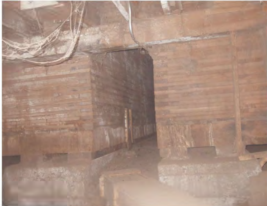
Grain bin walls in the basement
