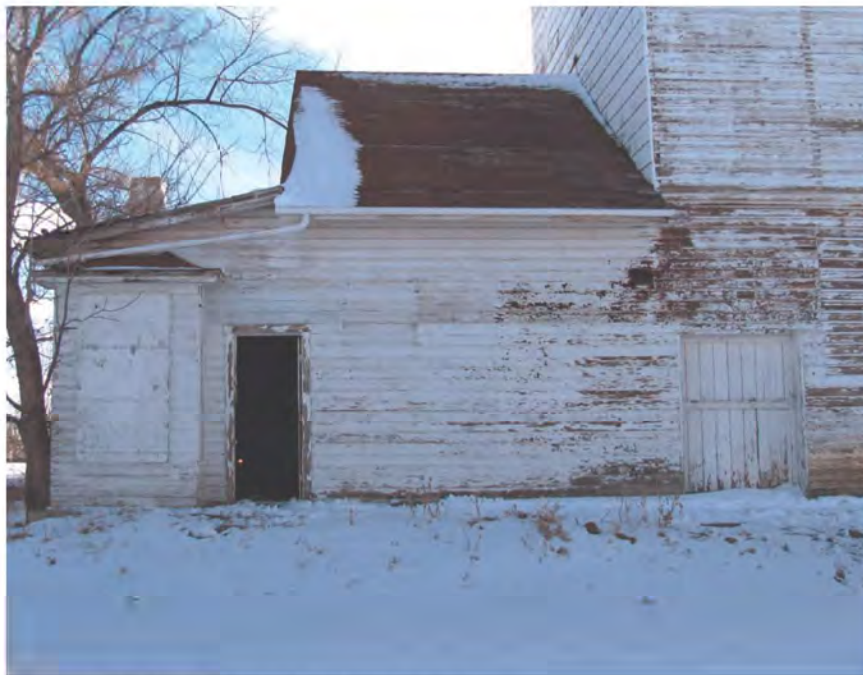
Window 1 and Doors 4 and 5 on the west elevation
