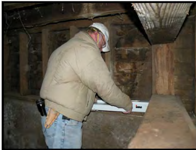
Figure 3. Resistance drilling a sill beam in the basement between Basement Storage and Tower Level 0.
