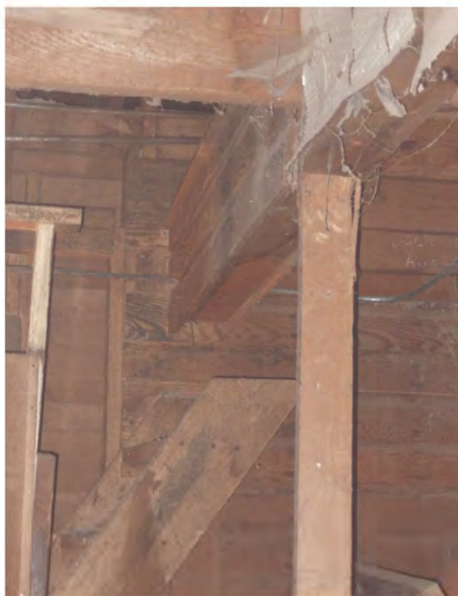
Section 2: Removed bearing wall supporting second floor framing with wood prop
