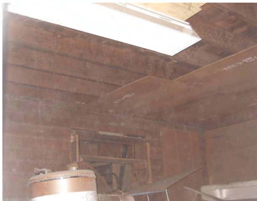
Section 2: West bay of second floor framing
