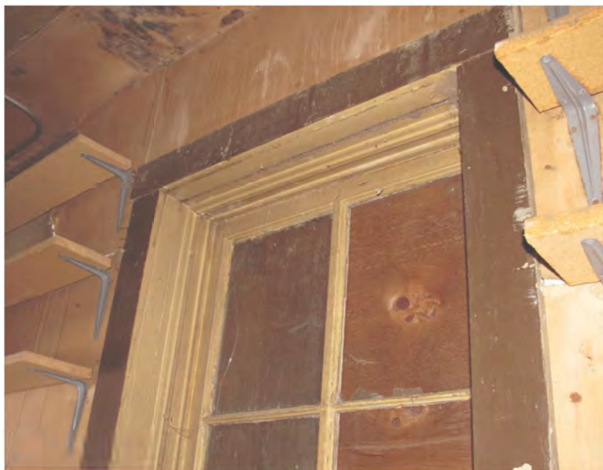
Window 7 frame detail
