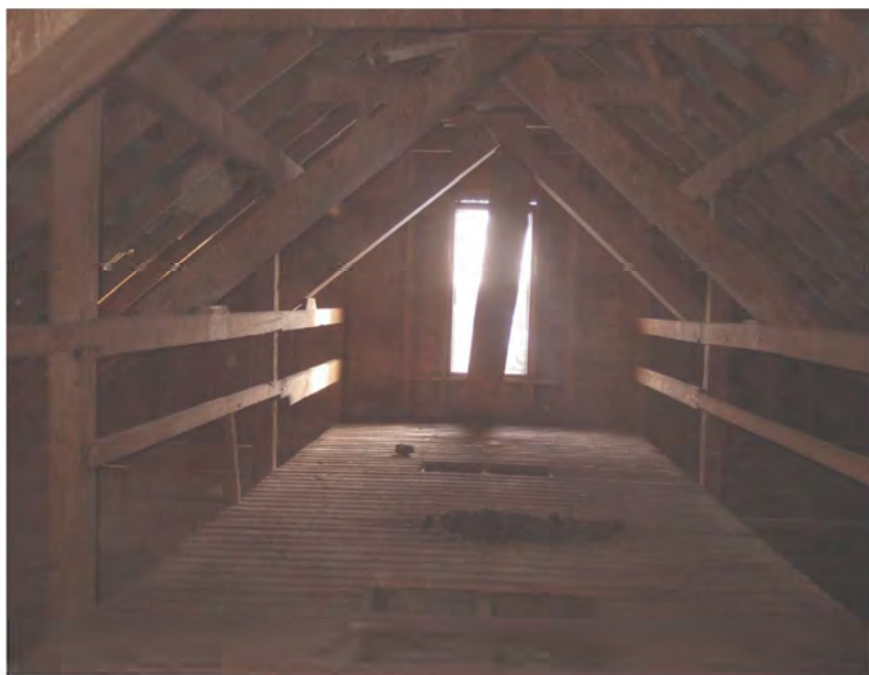
Section 4: Fifth floor framing, looking south
