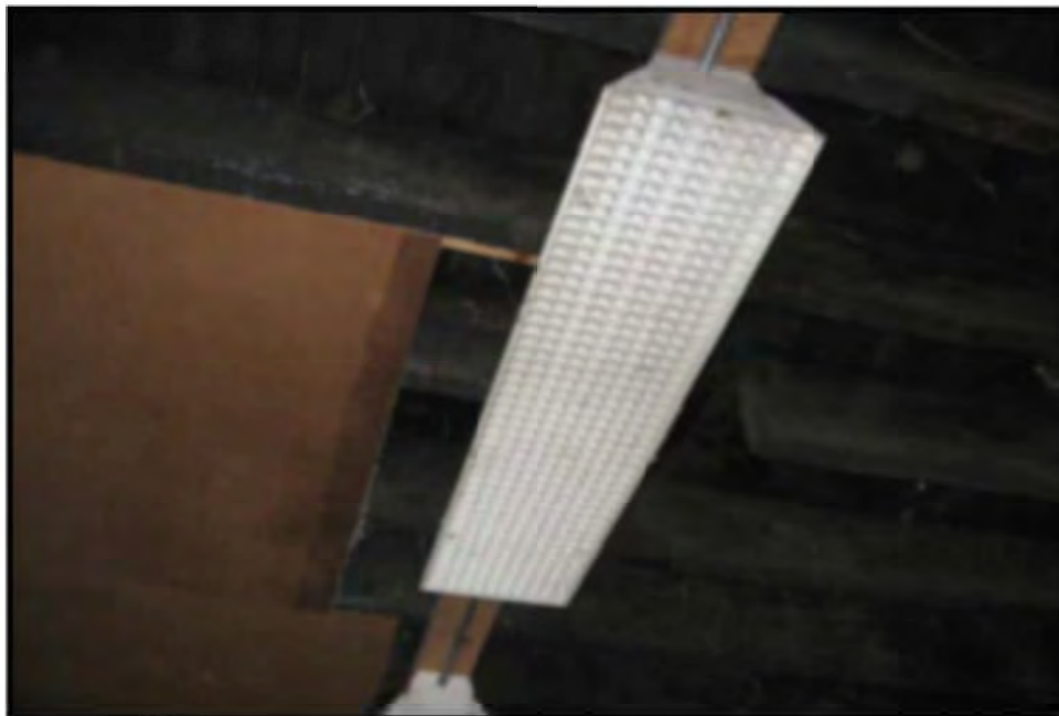
Photo 1 - First Floor Light Fixture
