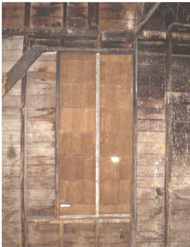
Window 12 interior side
