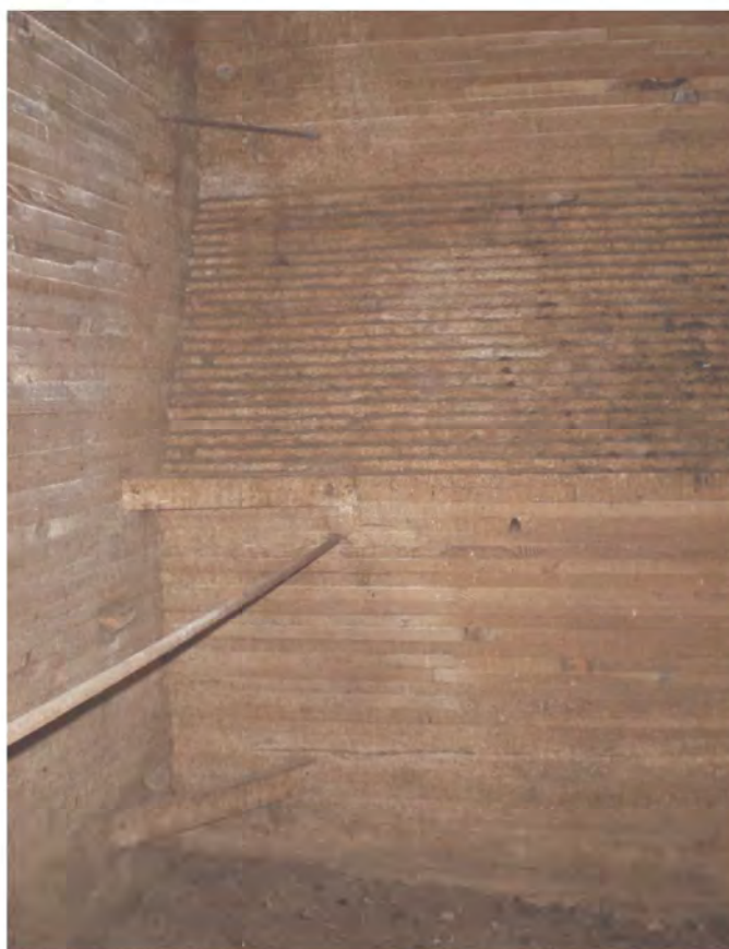
Fifth Floor - In Bin 5 looking east at stepped wall at bottom of bin
