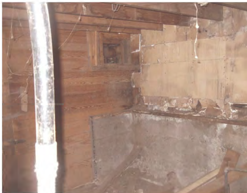
Section 1: Foundation wall at grid intersection Z/1
