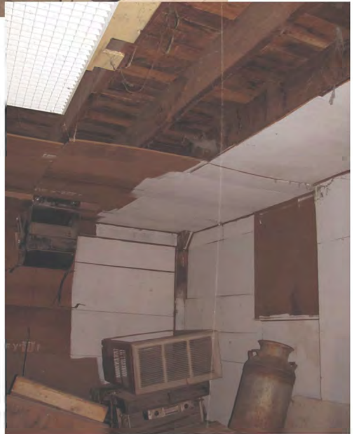
First Floor - Back Room various wall and ceiling finishes.
