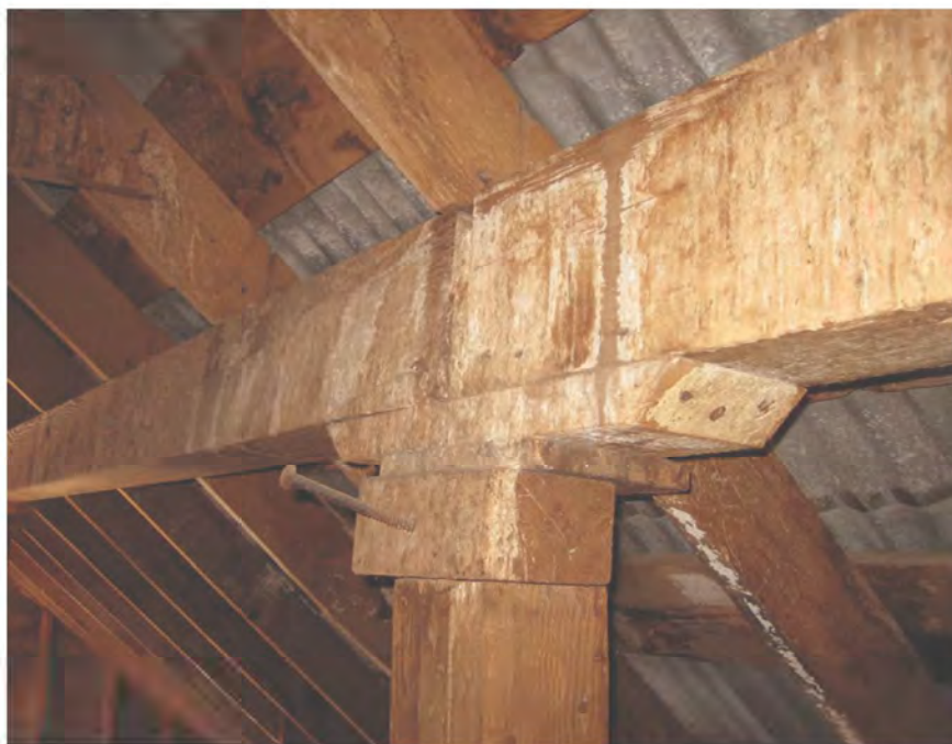
Stacked boards supporting roof structure
