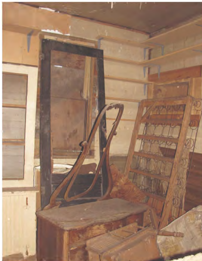
First Floor - Office north and east walls
