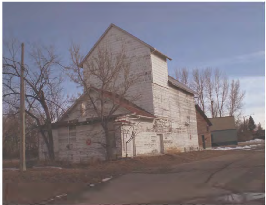
Electrical pole to the north and asphalt drive to the west of the Grain Elevator
