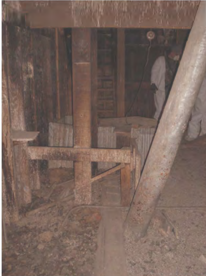
Fourth Floor - Chutes, original elevator track and corrugated metal over the stair
