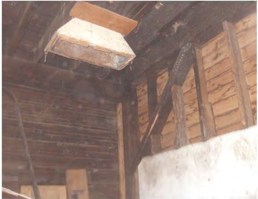
Section 3: First floor exterior wall along grid Z; stud infill at timber post and beam framing
