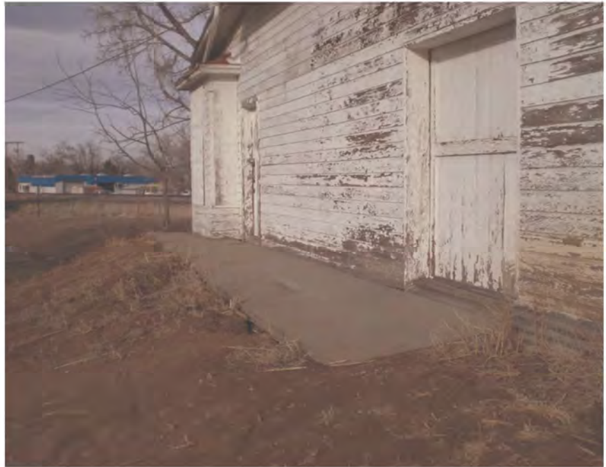
Section of the original wood walkway that remains on the west side of the building
