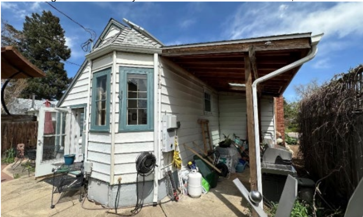
Recent images of 733 Mckinley from Historic Structure Assessment, 2024
