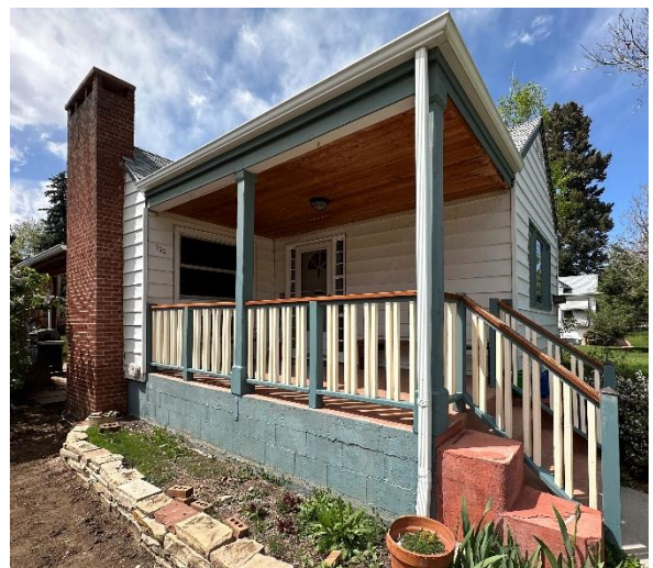
Covered front porch.
