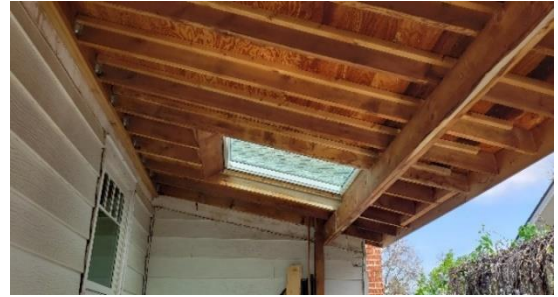
Southwest porch roof structure.
