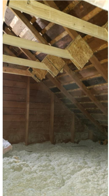
Original roof framing with newer collar ties.
