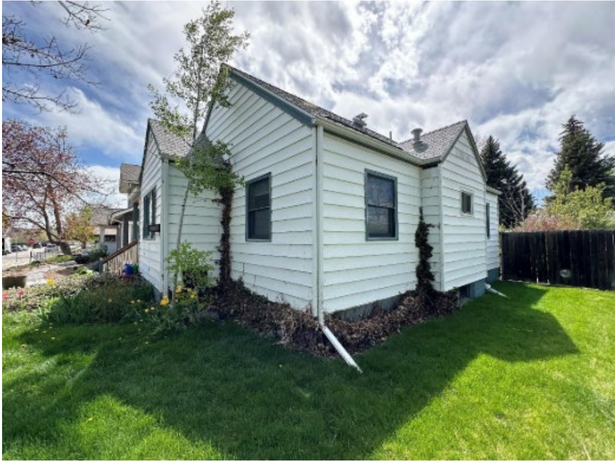
Recent images of 733 Mckinley from Historic Structure Assessment, 2024
