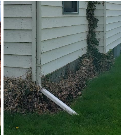
Grading and growth at the northeast corner.
