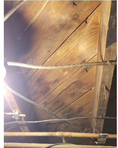
Original floor joists and sheathing.
