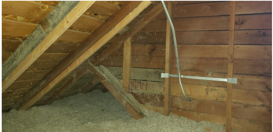
West gable showing gable end wall studs and original wood siding attached directly to the wall studs.
