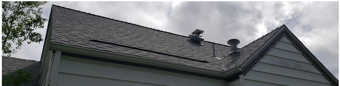
Asphalt composition shingle roof, ridge vents, and low roof shingle vents.
