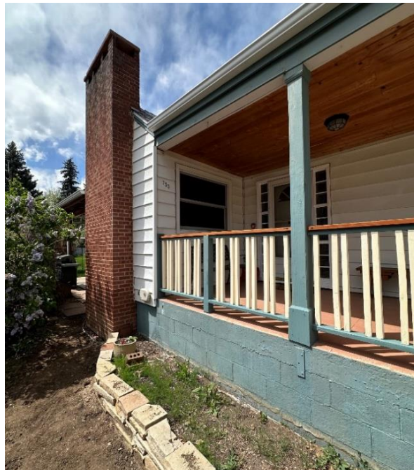
CMU porch foundation.
