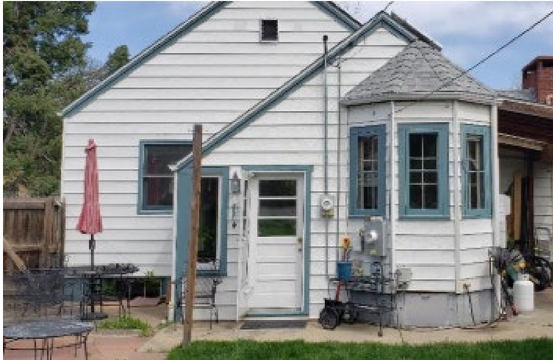
Recent photo highlighting concrete apron from Historic Structure Assessment, 2024
