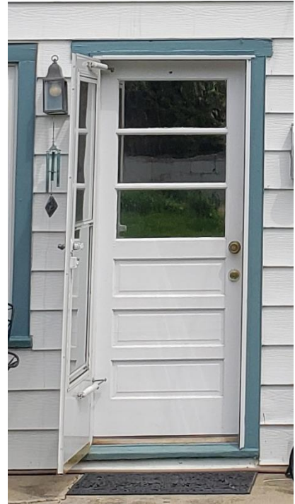
Rear door and light fixture
