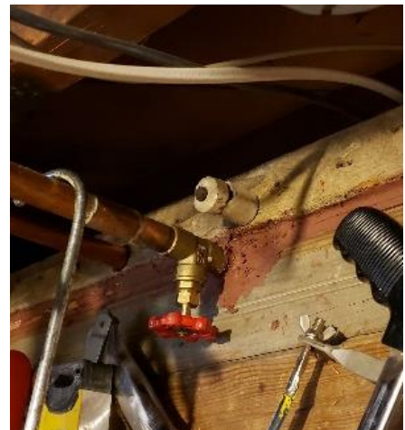
Romex wiring with knob and tube remnants.
