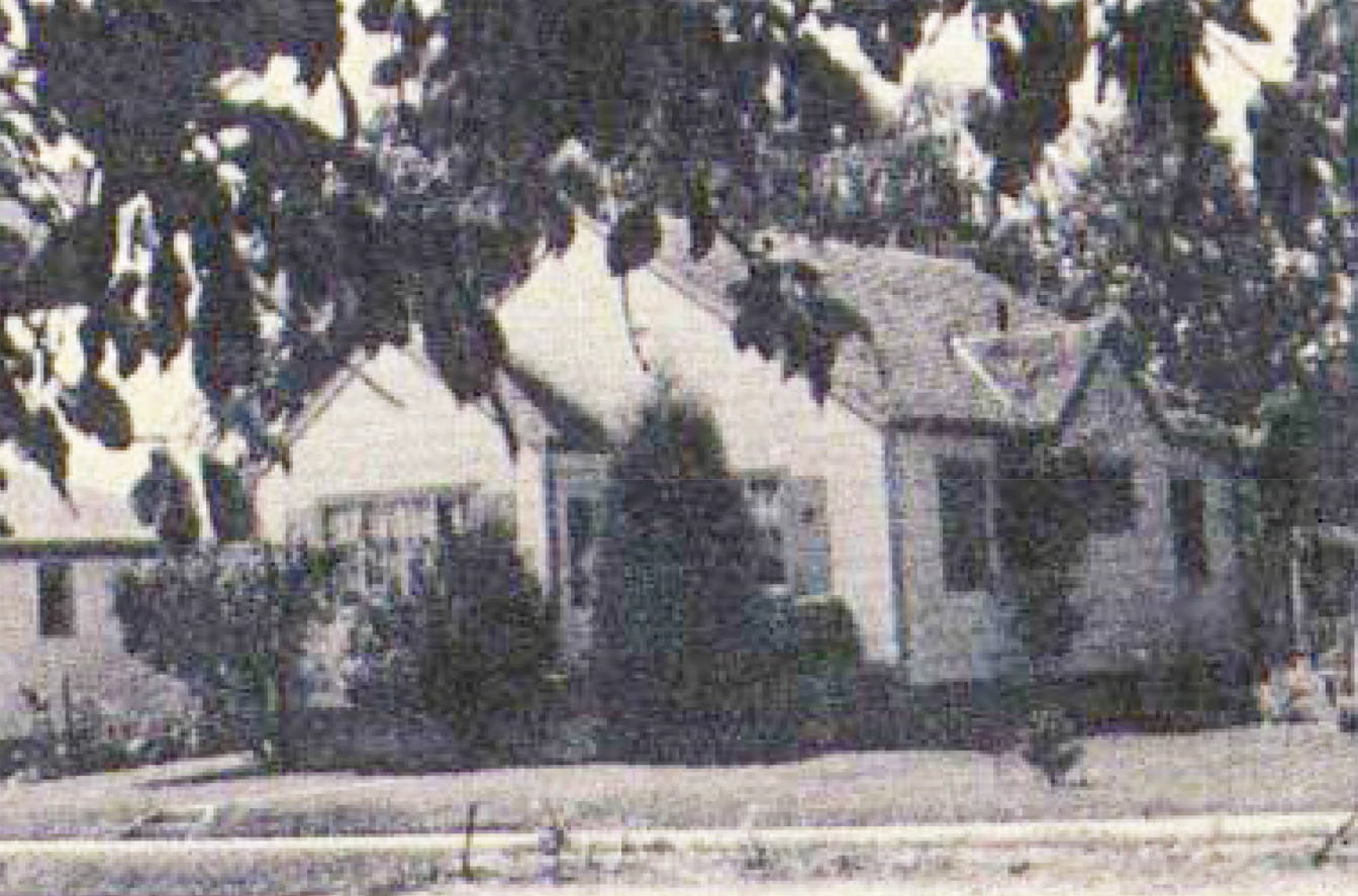
1948 PHOTO OF 733 MCKINLEY AVE.
