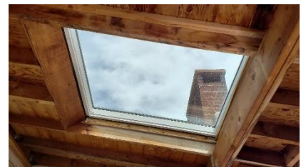
South facing skylight in patio roof.
