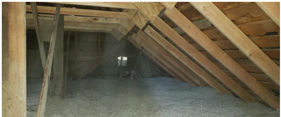
Roof bracing of the ridge beam and rafters, attic insulation throughout.
