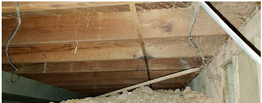
Floor framing in the crawlspace.
