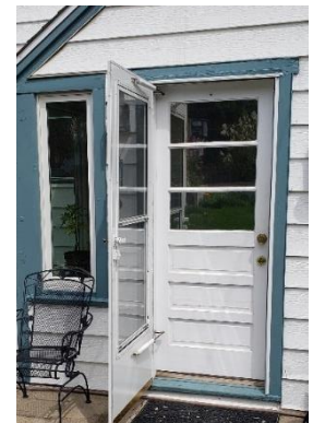
Rear door and storm door.
