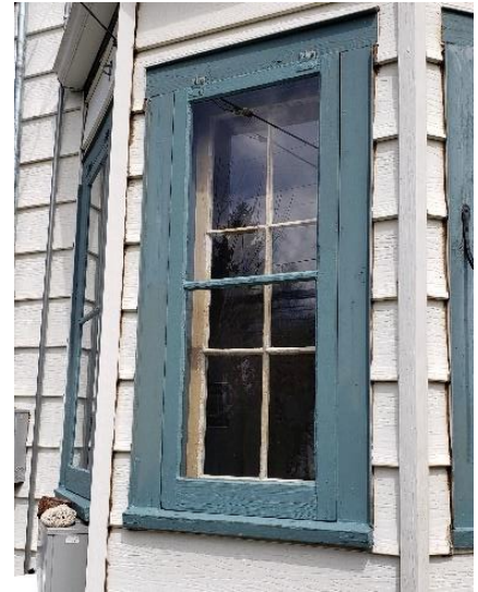
Bay window and storm window.
