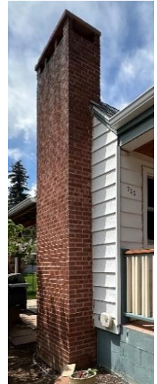
South addition chimney.
