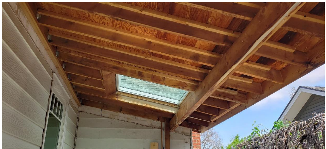
Exposed roof structure of the south side covered patio.
