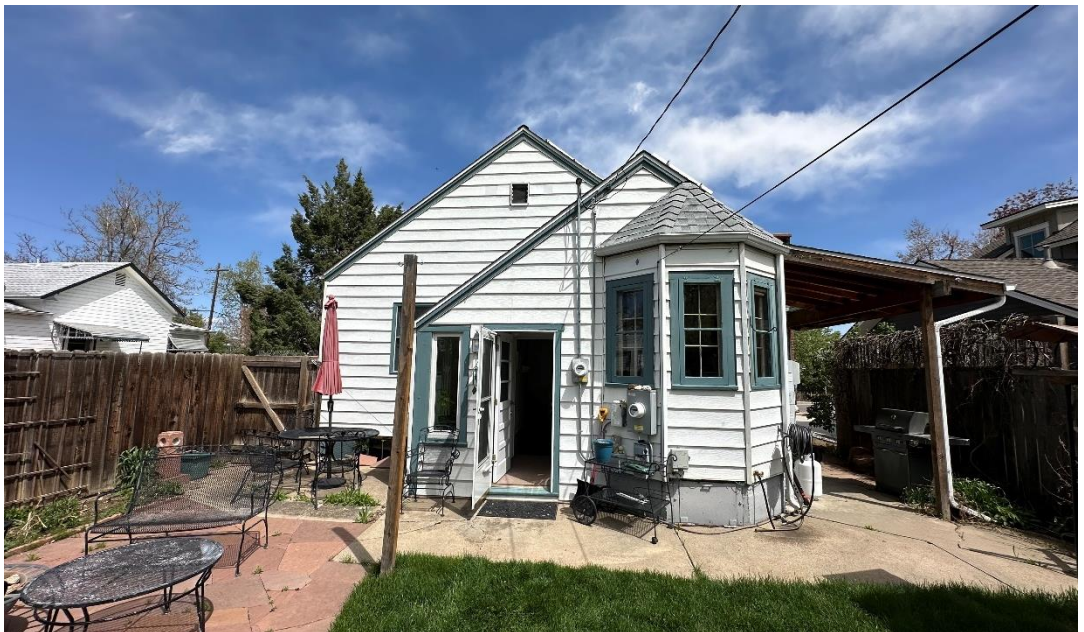
2024 Rear Façade, Looking East.
