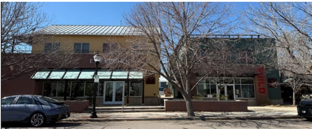
Housing over retail on Main Street (12-24 DU/acre)
