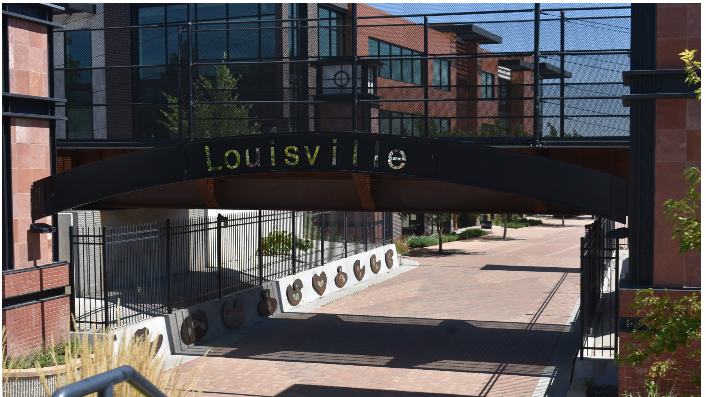
Louisville Bridge Source: DesignWorkshop
