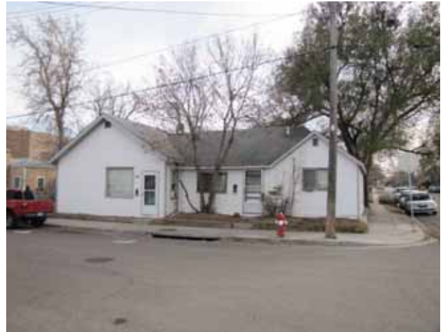
800 Spruce: Louisville Times Office Wood frame cross gable
