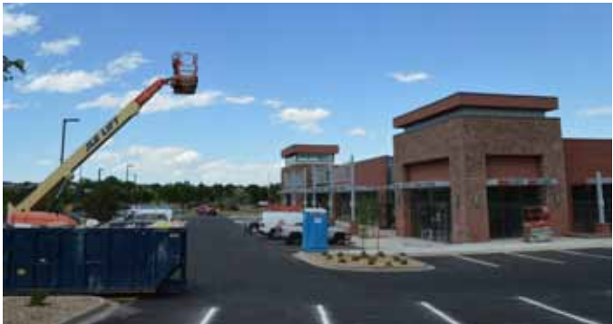
Construction of McCaslin Marketplace
